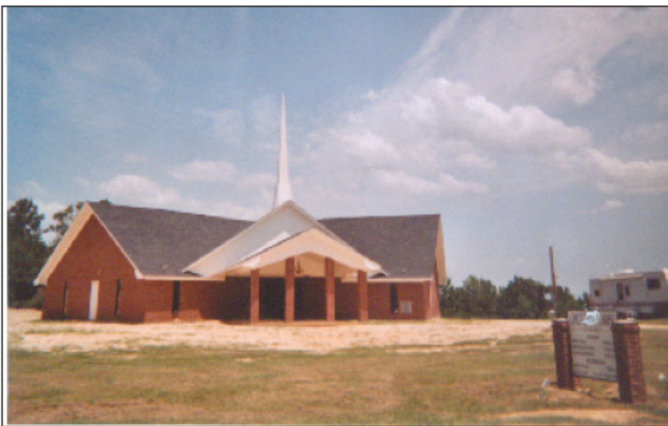
The newly constructed Anadarko Church of Christ building is now complete.
