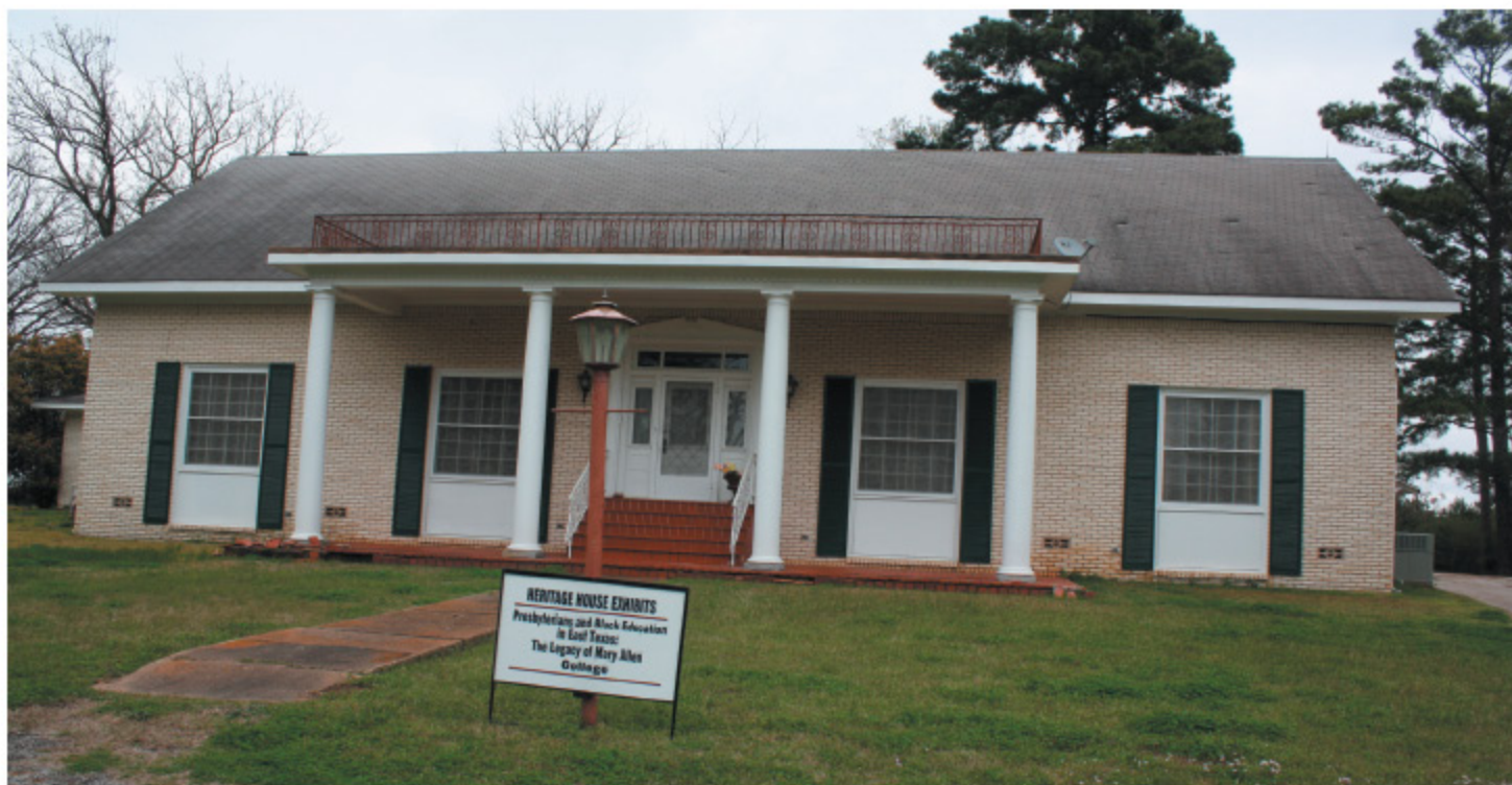
Mary Allen Heritage House Office and Collections Center located at 1503 South 4th Street, Crockett, TX.
