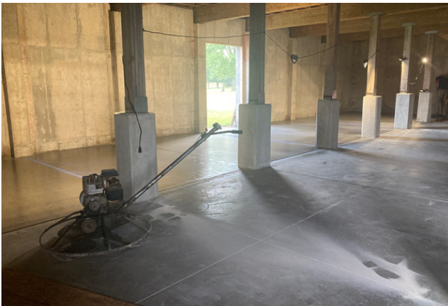
Above left: The Piatt County Museum barn as it stands at #1 Heritage Lane. Below Left: The concrete floor being finished in the barn. Right: The upper story of the barn. Long-term plans are to completely finish the interior of the structure to allow for the site to be used for display, educational and meeting space.
