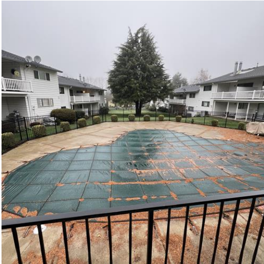
Description: Replacement of the pool cover.
