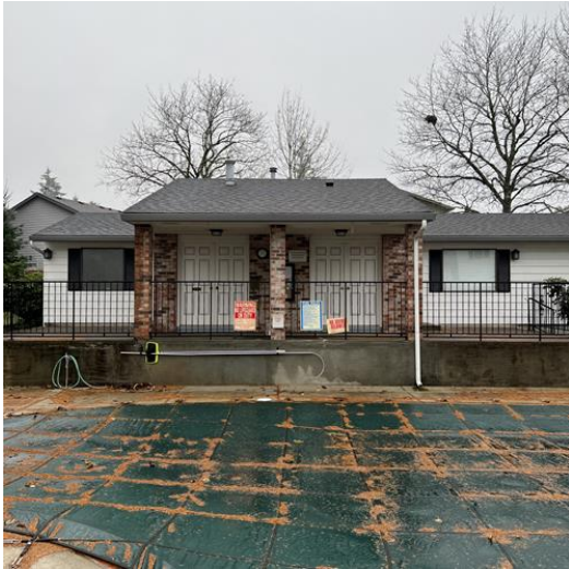
Description: Replacement of the utility pump room doors.
