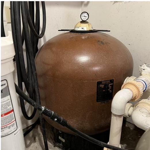
Description: Replacement of the pool sand filter in the pool equipment room.
