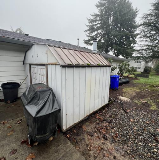
Description: Replacement of the 8' x 10' metal maintenance shed behind the clubhouse.
