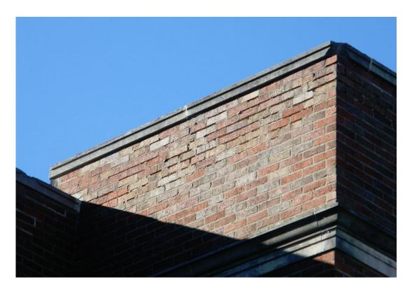
Parapets exhibited signs of cracked, loose and missing mortar. Some parapets leaned slightly inward but seemed to be firmly attached to the walls below. There is moisture infiltration in the parapet walls.
