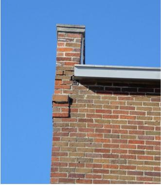
Parapets are generally two wythe and three wythe walls with heights less than 24 inches above the roof.
