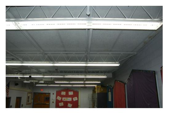
Tectum deck on steel joists on concrete masonry walls. Bob Hoyt noted that the roof on this 1964 building leaked.
