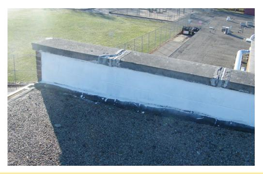
Cracked and damaged joint sealant between the coping stones is allowing water infiltration into the wall
