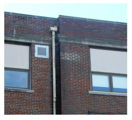
The faulty scupper and downspout is allowing water to enter the building through the wall at rooms 302 and 202 and below.
