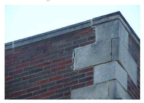
Cracked and missing mortar in the parapet walls allows moisture to enter the building. Displaced brick and stones as here on the northwest corner should be repaired or secured as soon as possible to prevent falling debris.
