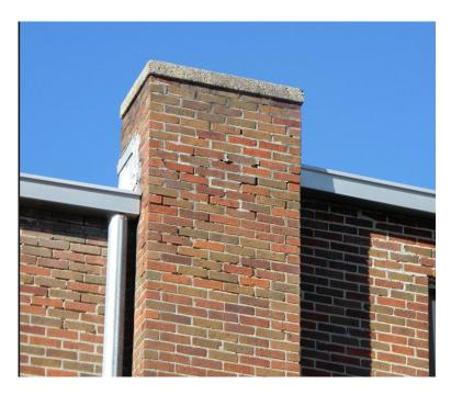
Cracked, loose and missing mortar allows moisture to infiltrate the building.
