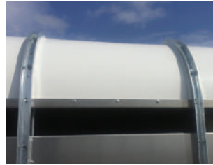
Aluminium spouting reinforces the roof.
