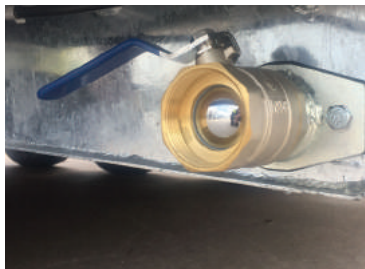
Collection tank— fully welded and sealed —hygienic disposal.
