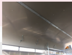
Tough central roof structure with edge retainer.
