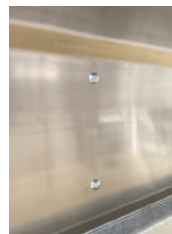
Mono bolts pin and collared joint fabrication.
