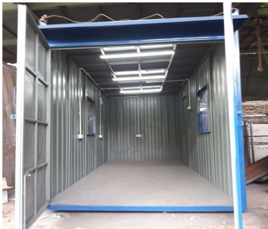
Checkered plate flooring
