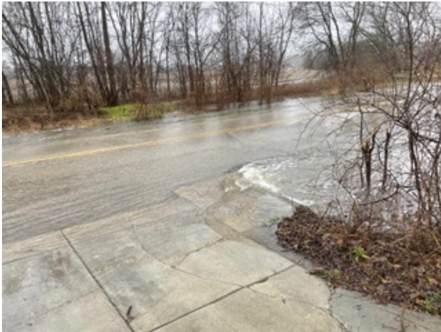
Photo 3: Town Line Road flooding — additional view showing extent of road inundation and standing water in surrounding area.
