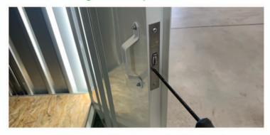
**1.27** Finally adjust the ball catch using the Philips screwdriver so that the door closes easily but remains in position when unlocked. Clockwise brings the ball out and anti-clockwise pushes it in again.
