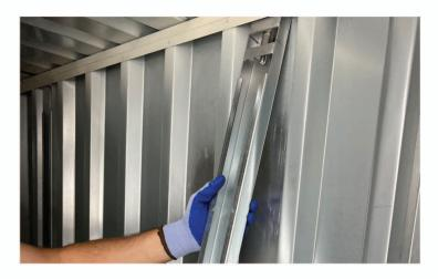
**3.1** Insert the top of the shelf upright into the top rail of the flat pack container, these should be positioned so that the shelf will be stable and secure when loaded. Not too close to the end and wide enough apart that the shelf will be balanced. Make sure that the shelf upright is now located behind the bottom rail of the container.
