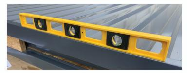
**1.14** If you need to move the parts to a new location, do so now. Begin with the base which needs to be level (check with the level), before starting the erection process.
