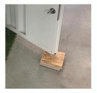
**1.18** Now unlock the door and prop it open using the wooden packaging that you removed earlier. If you are erecting on an exposed site, you may need others to hold the door panel to prevent it falling and causing damage.
