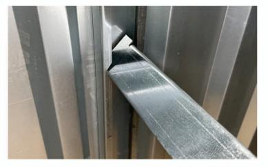
**3.4** Final position of shelf arm, when correctly fitted.
