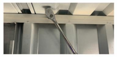
**1.24** Now fit the M8 bolts, nuts and two washers to secure the roof to the respective wall panels.
