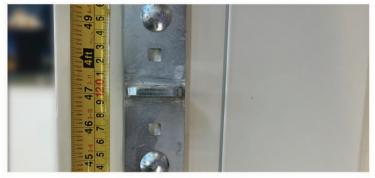
**3.1** For extra security its possible to fit more than one locking bar.
