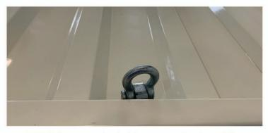
**1.25** Using your stepladder, access the top of the roof to screw in the 4x lifting eyes.
