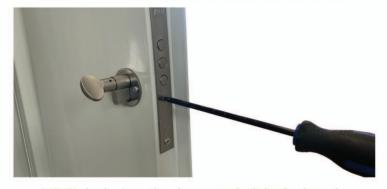
**1.17** Fit locks into the door panel, slide the barrels into the door and turn. Once the lock turns, this shows it is located correctly and the screw can be inserted and tightened using your Philips screwdriver.
