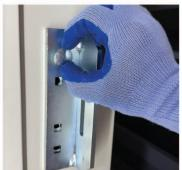
**3.6** Fit security plates using coach bolts provided (nuts on inside).
