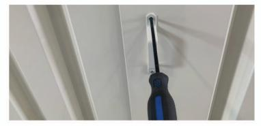
**1.26** Fit the handles onto the inside and outside of the door using the screws provided.
