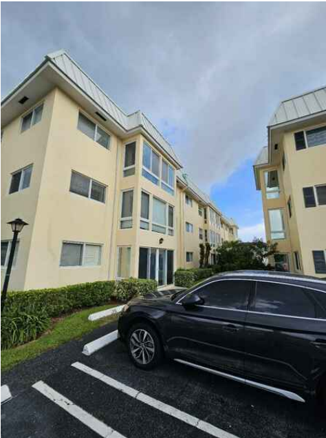
rear elevation of building
