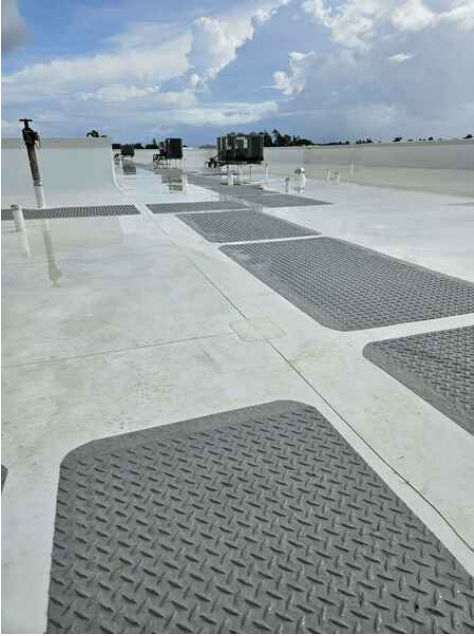
roof elevation pic # 1
