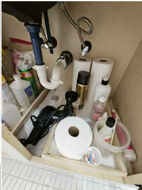
guest under sink plumbing
