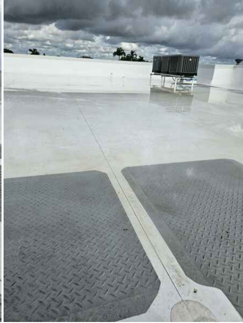
roof elevation pic # 2
