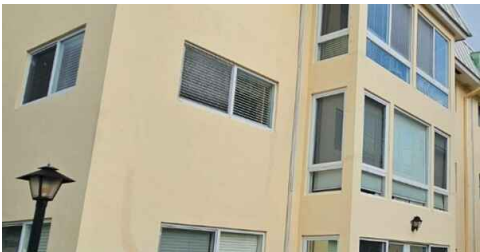
rear elevation of unit
