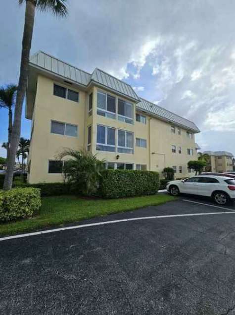
right elevation of building
