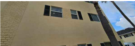
side elevation of unit
