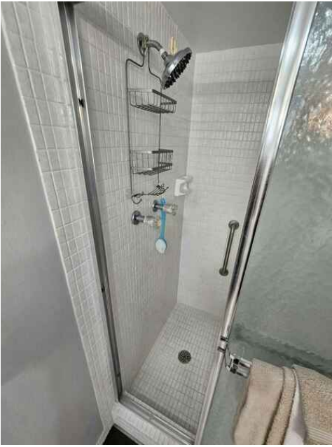
guest shower valves and drain
