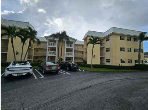
front elevation of building
