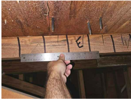
4 inch nail spacing roof deck attachment
