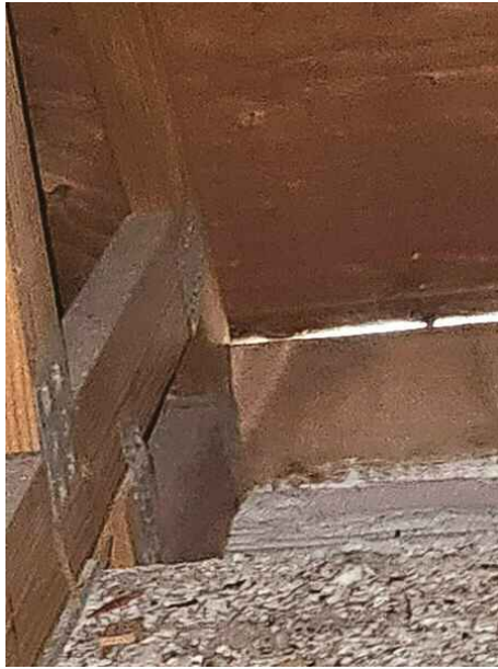
toe nails roof to wall attachment
