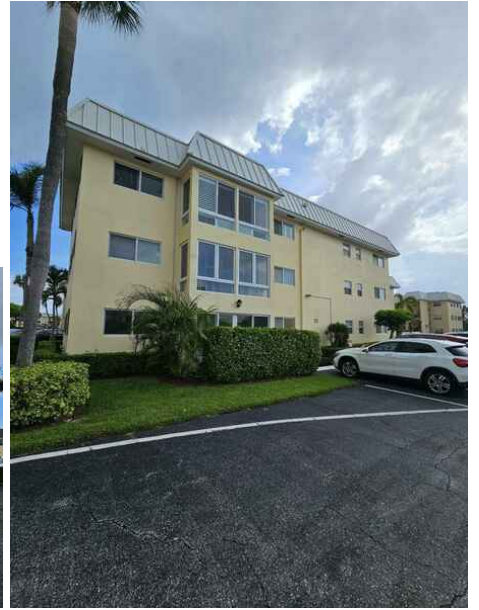
right elevation of building
