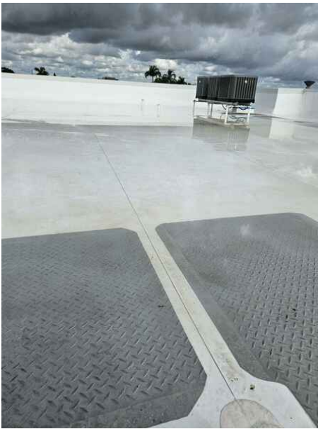
roof elevation pic # 2
