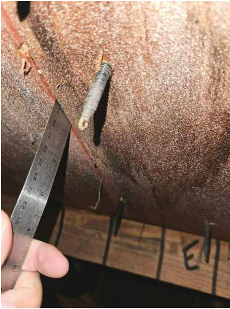
7/16 inch roof deck thickness
