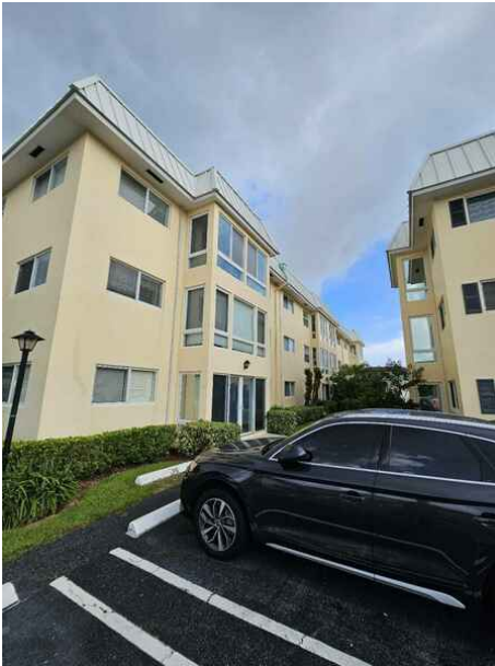
rear elevation of building
