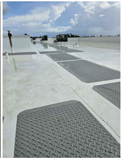
roof elevation pic # 1
