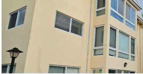
rear elevation of unit
