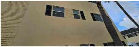
side elevation of unit
