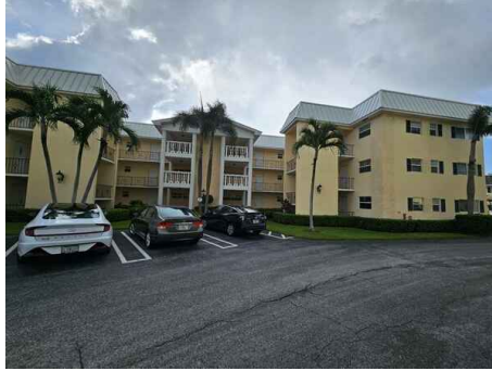
front elevation of building
