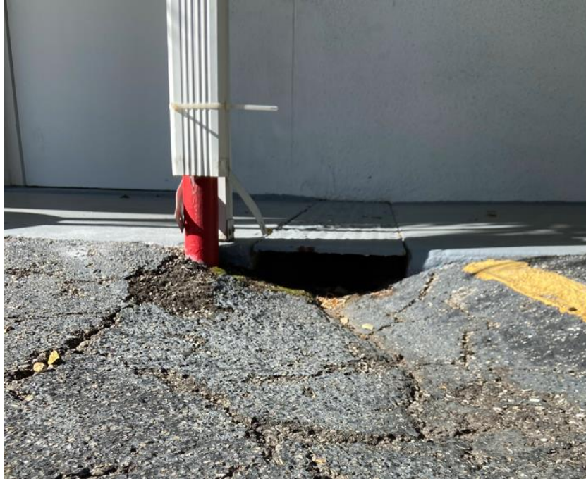
Figure 17: Outfall for roof drain at farthest North side
