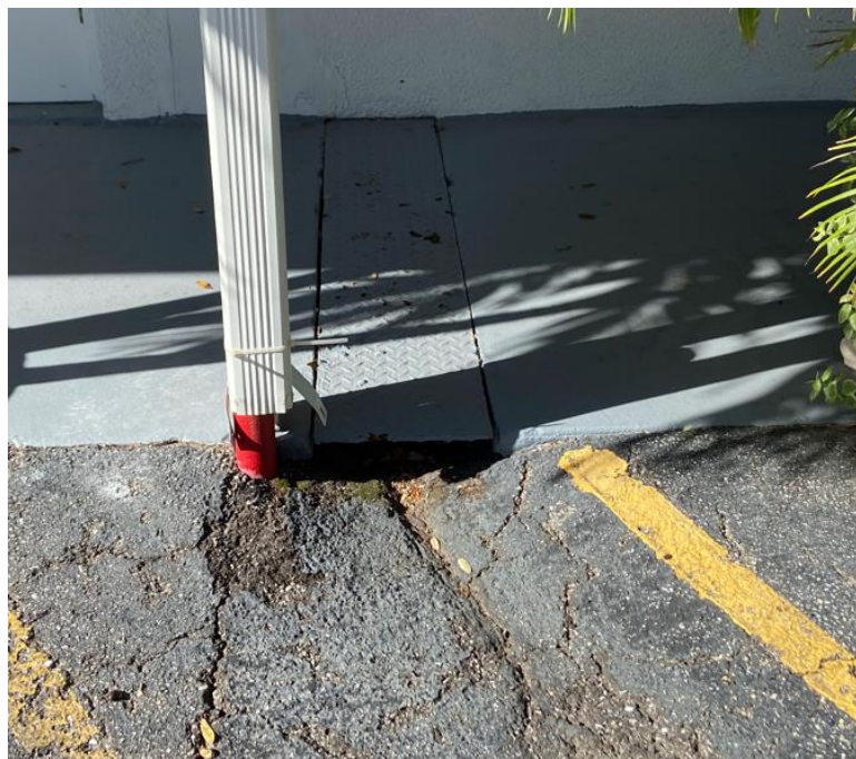
Figure 16: Outfall for roof drain North of entrance
