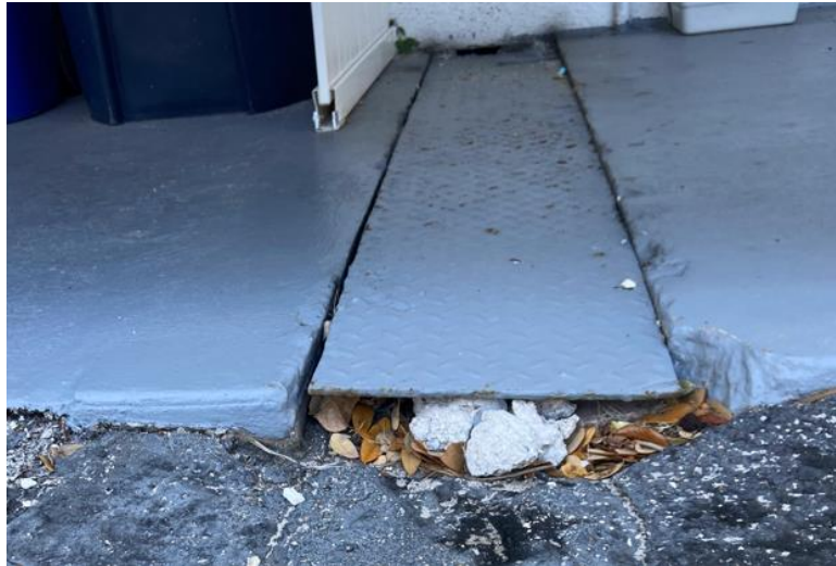
Figure 15: Outfall for South roof drain
