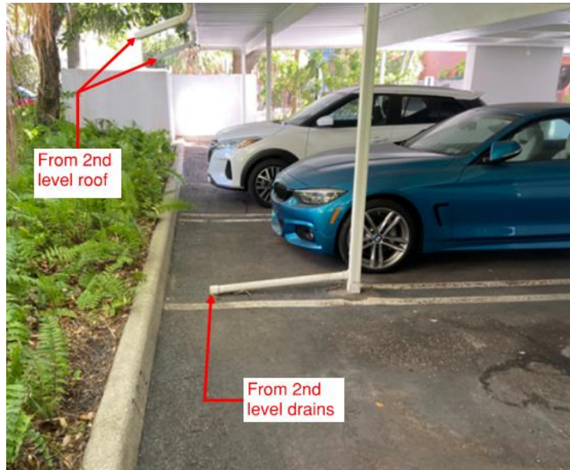
Figure 18: Upper-level drainage discharge (North of site)
