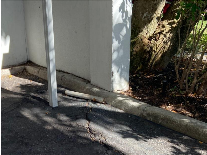
Figure 10: Cracked curbs.
