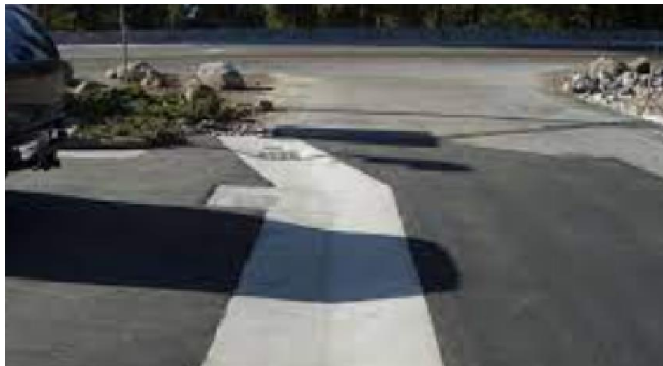
Figure 24: Paved Swale in Concrete
