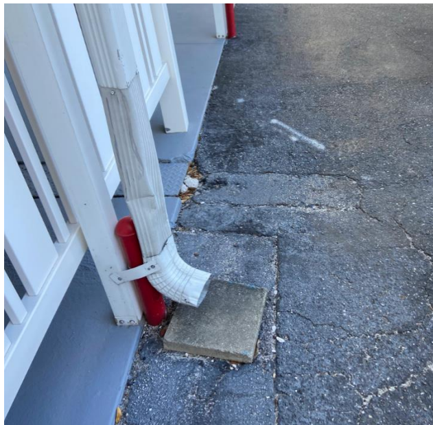
Figure 12: Downspout for small roof covering pedestrian path
