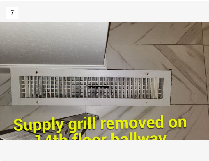
Project: Royal St. Andrews Association Date: 11/27/2023, 9:50am Creator: Jamie Vass
