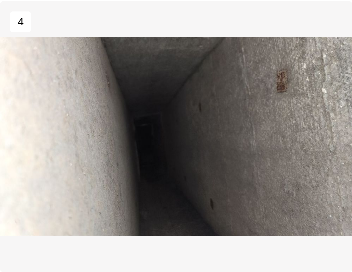
Project: Royal St. Andrews Association Date: 11/27/2023, 9:39am Creator: Jamie Vass
