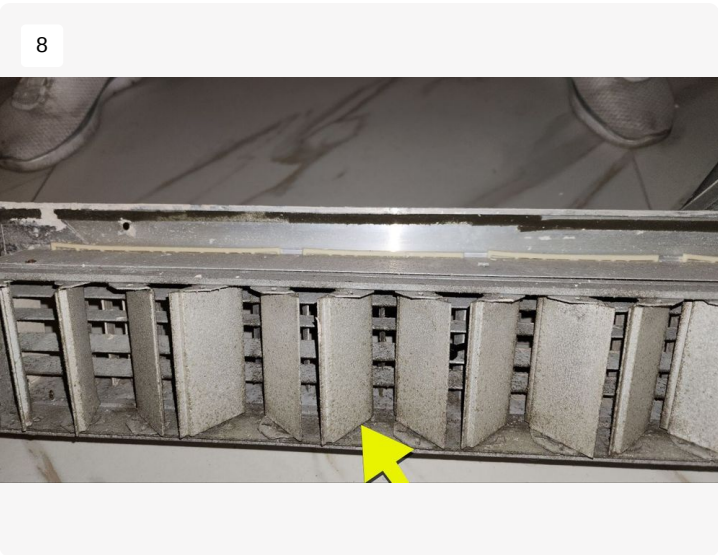
Project: Royal St. Andrews Association Date: 11/27/2023, 9:51am Creator: Jamie Vass
