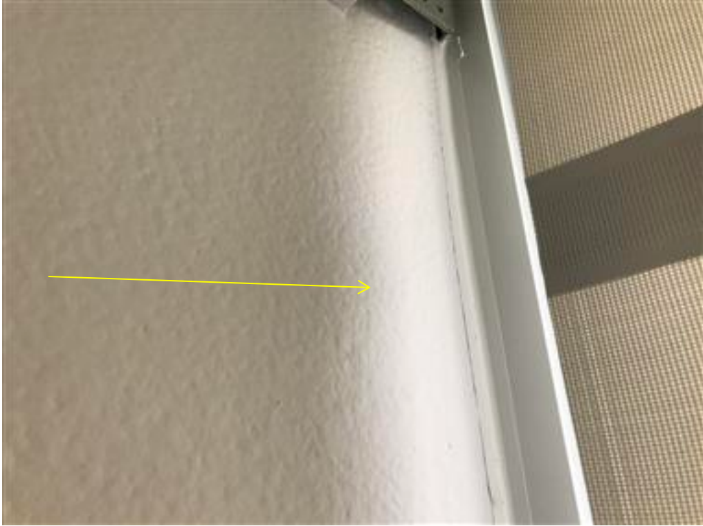
Photo 100-802, unfamiliar joint at SGD
