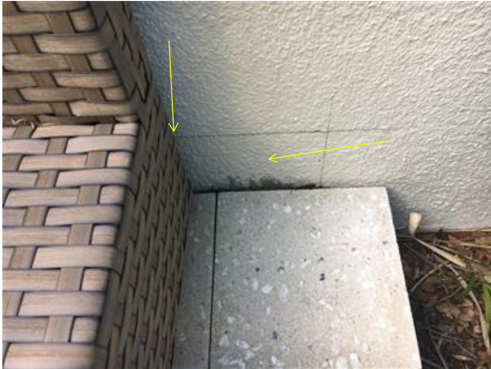
Photo 182-EXTERIOR, stucco cracks
