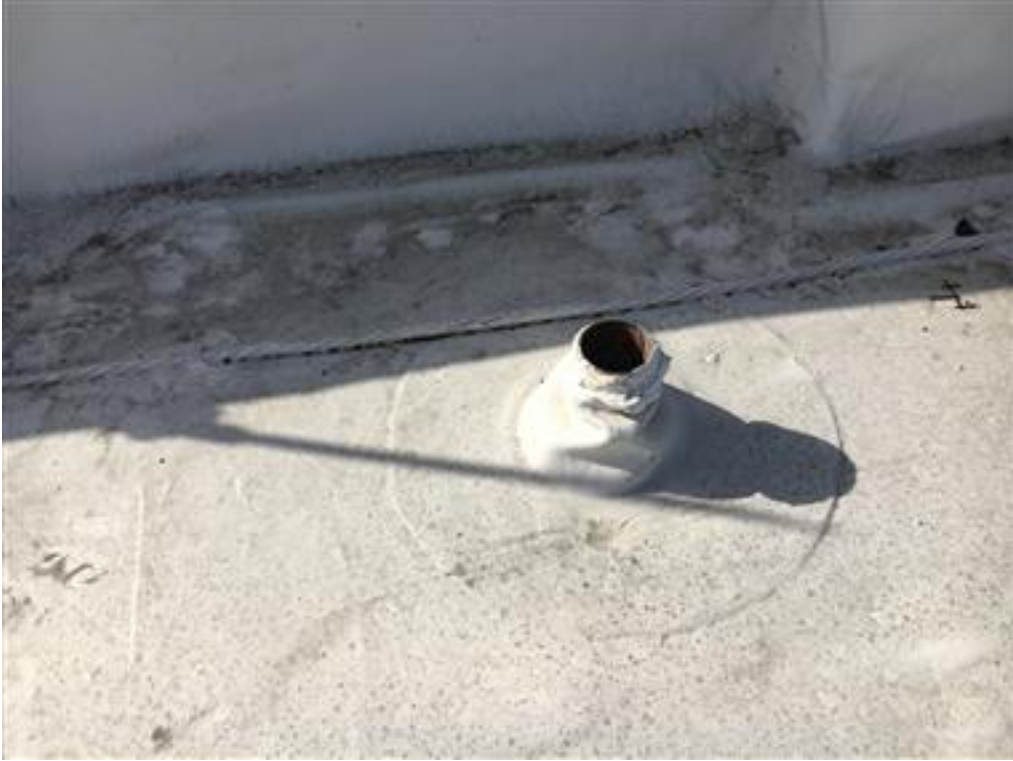
Photo 25-Typical vent stack
