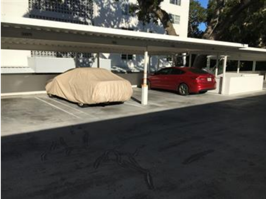
Photo 9-UPPER LEVEL WALLS- TYPICAL
