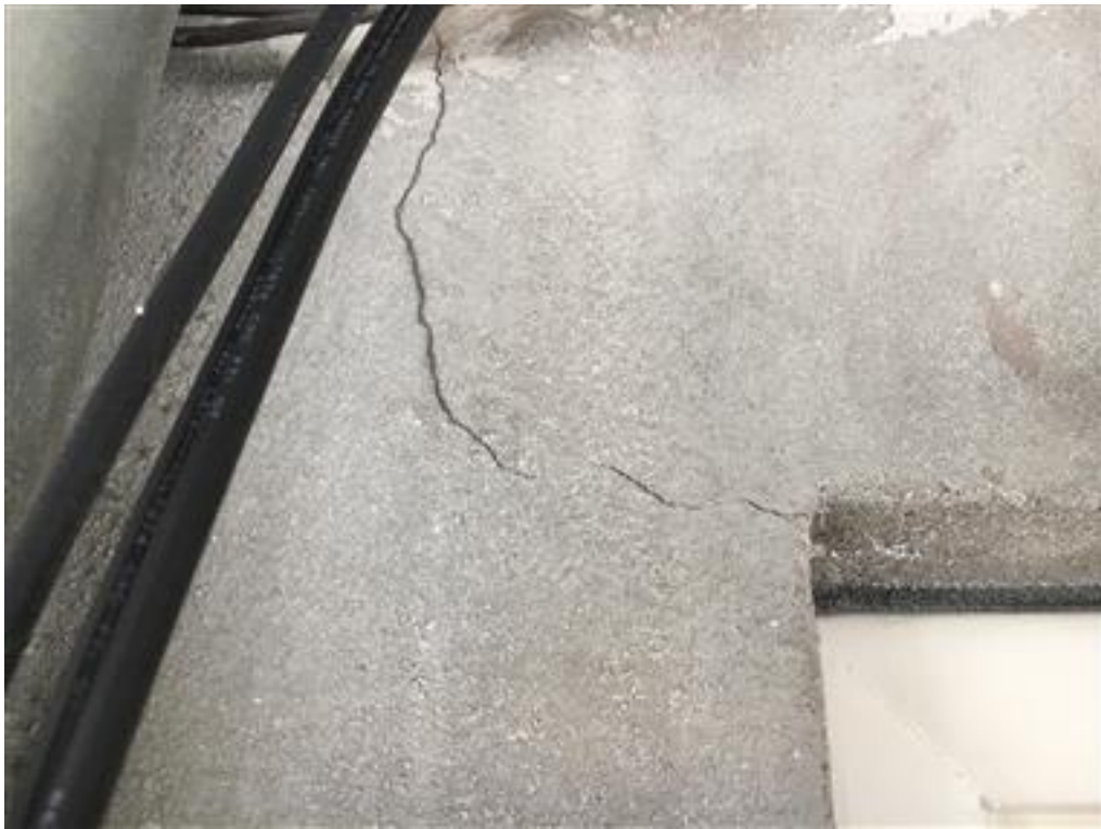
Photo 28-5 TH FLOOR- HLC
