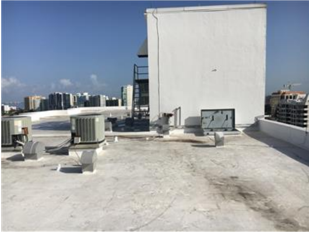
Photo 3-General view, elevator penthouse
