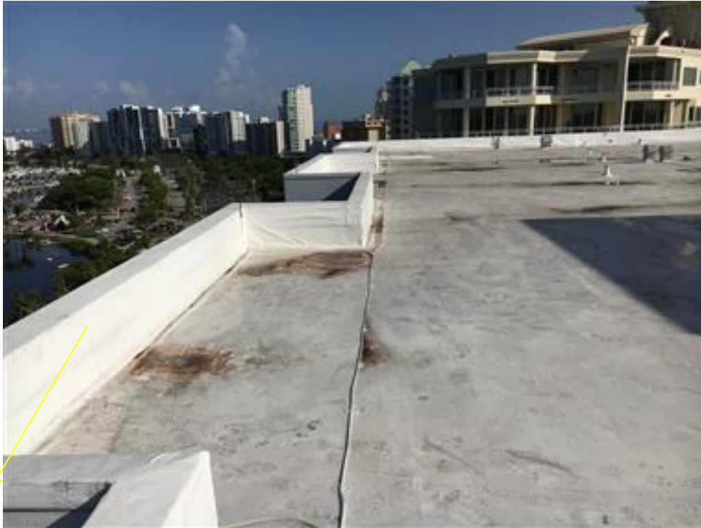
Photo 29-General view of coping detail, wrap over
