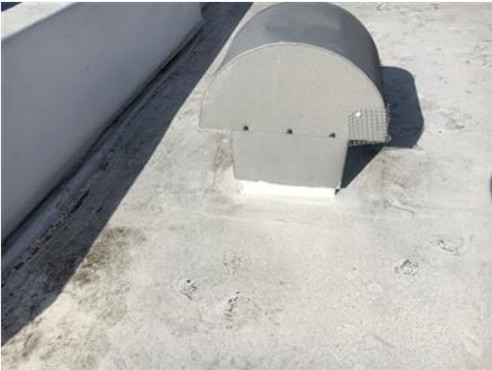
Photo 26-Typical vent hood
