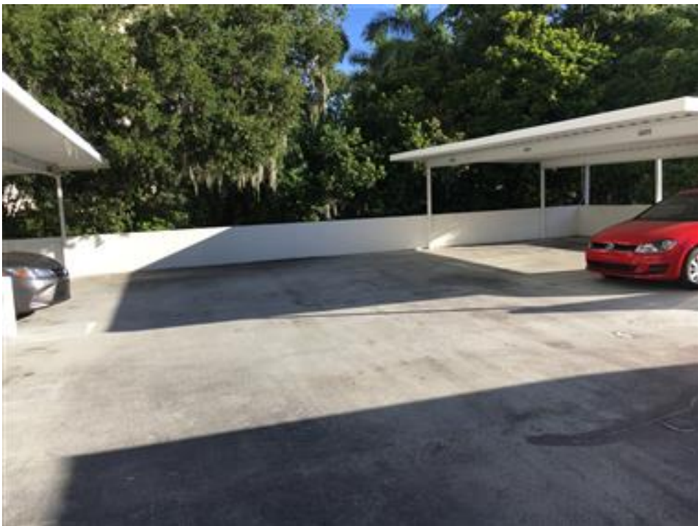
Photo 10-UPPER LEVEL WALLS- TYPICAL
