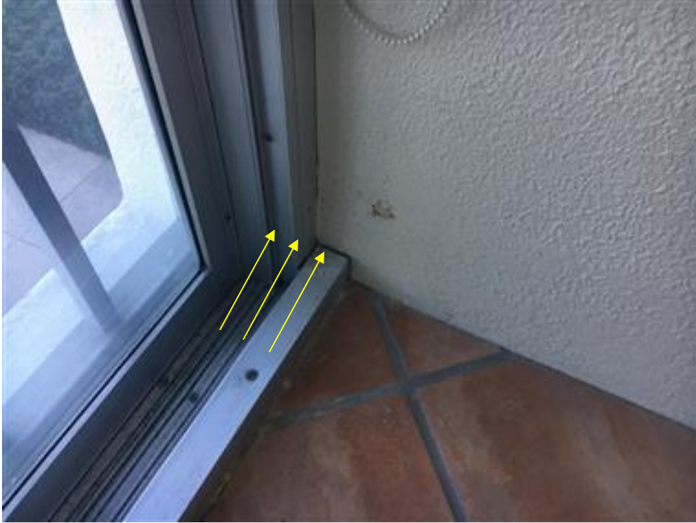
Photo 176-Unit 304, peeling paint
