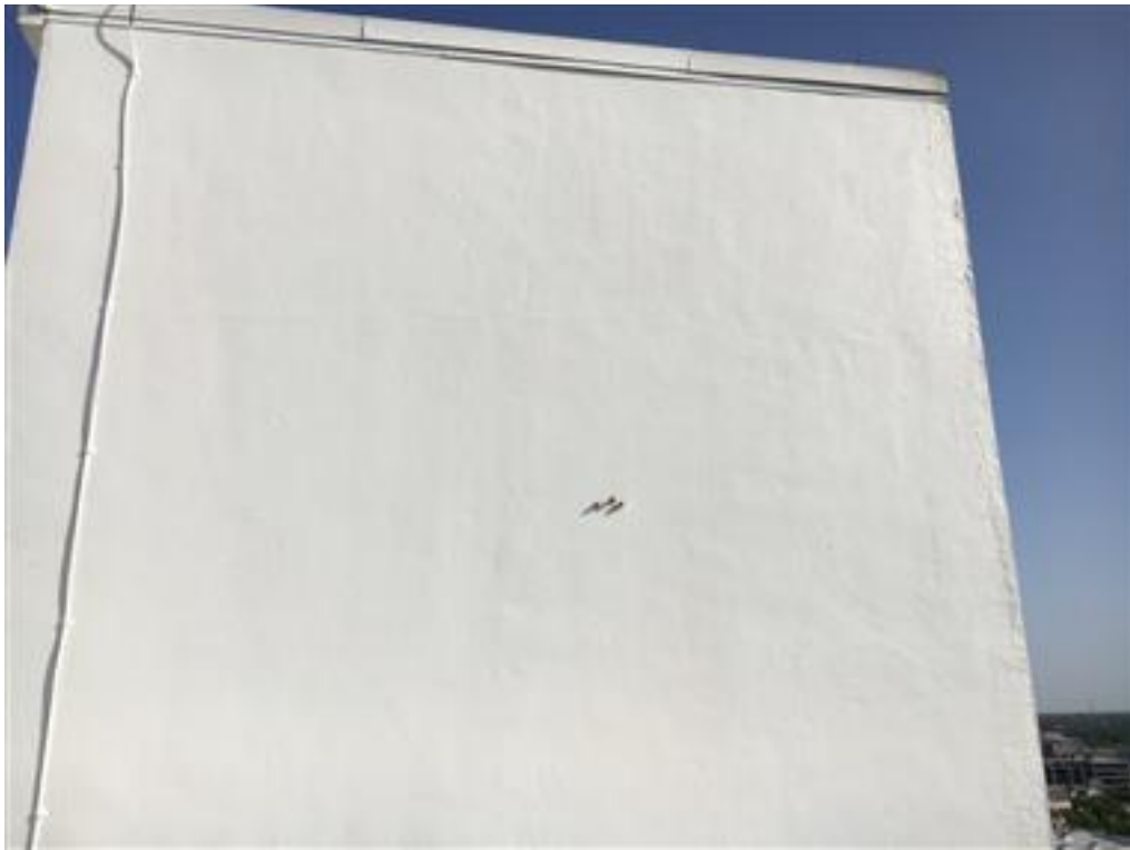
Photo 22-Elevator penthouse, good condition, south
