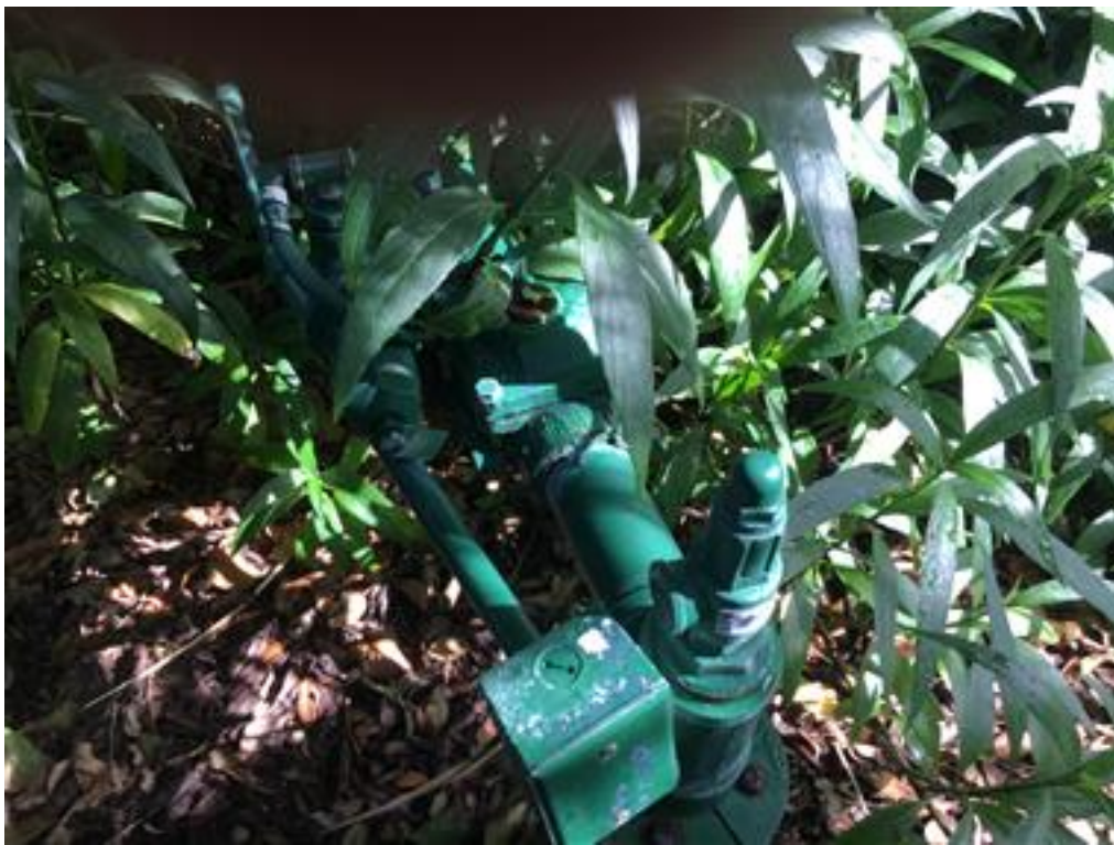
Photo 4- Irrigation well, good condition
