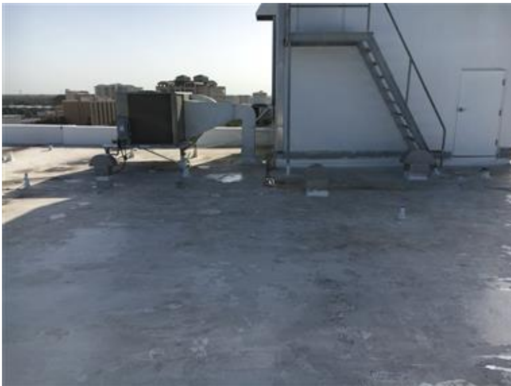
Photo 6-General view, elevator penthouse
