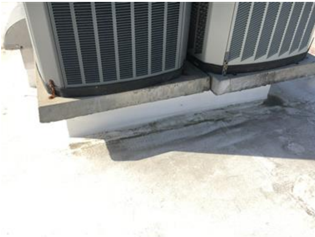
Photo 38-Typical AC mounting-curb
