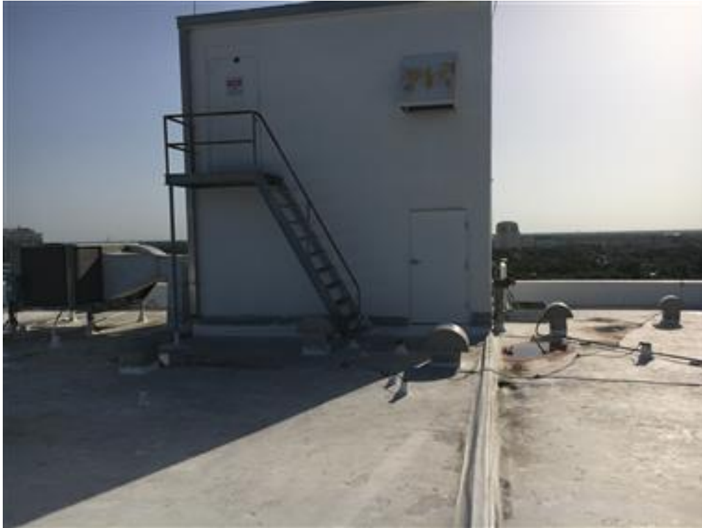
Photo 5-General view, elevator penthouse
