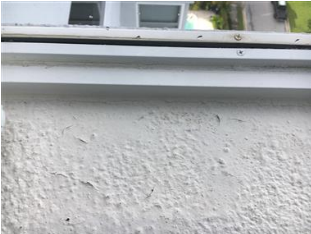
Photo 14-Unit 1502, blistering paint
