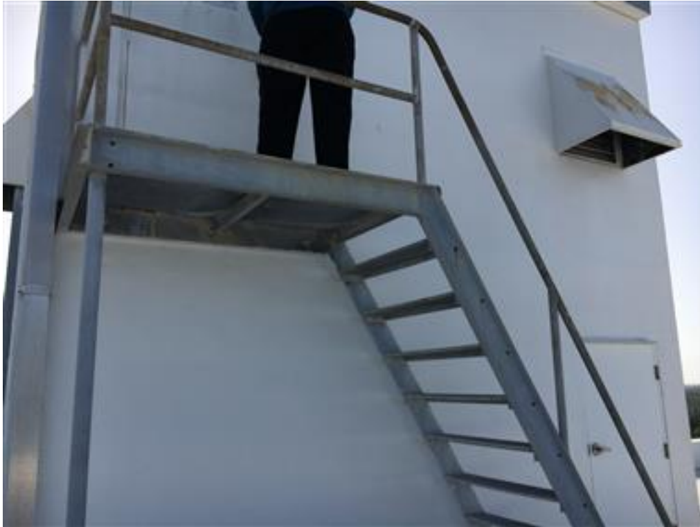
Photo 19-Elevator penthouse, good condition, west
