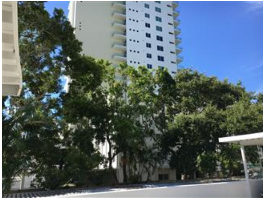
Photo 1- AREA BY SOUTH BOUNDARY
