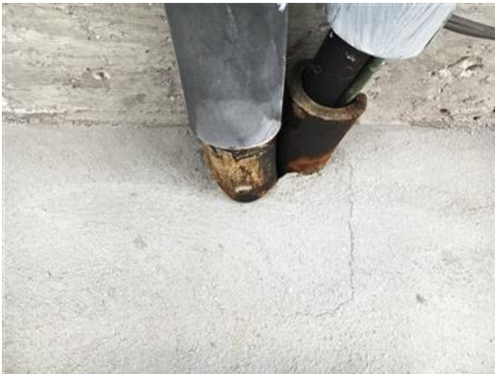
Photo 29-5 th FLOOR – HLC
