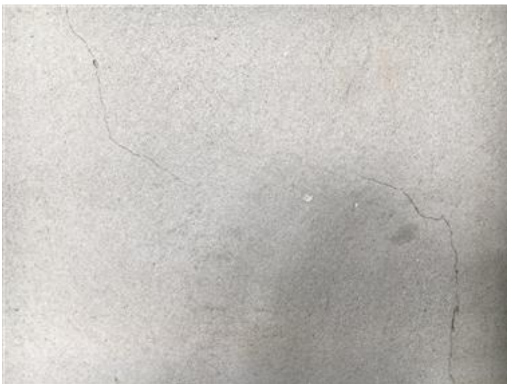
Photo 30-5 th FLOOR- HLC
