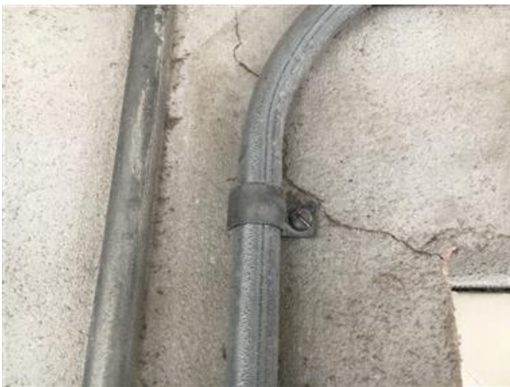
Photo 10-11 th FLOOR- HLC
