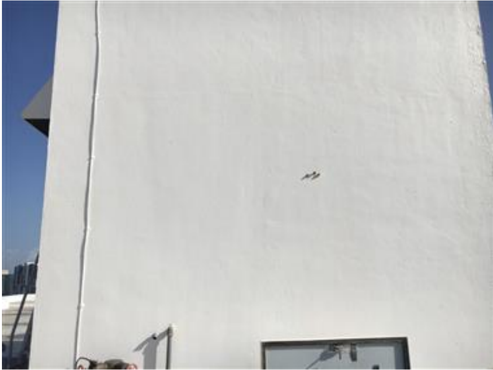
Photo 21-Elevator penthouse, good condition, south
