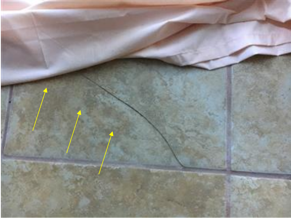
Photo 168-Unit 204, cracked tile
