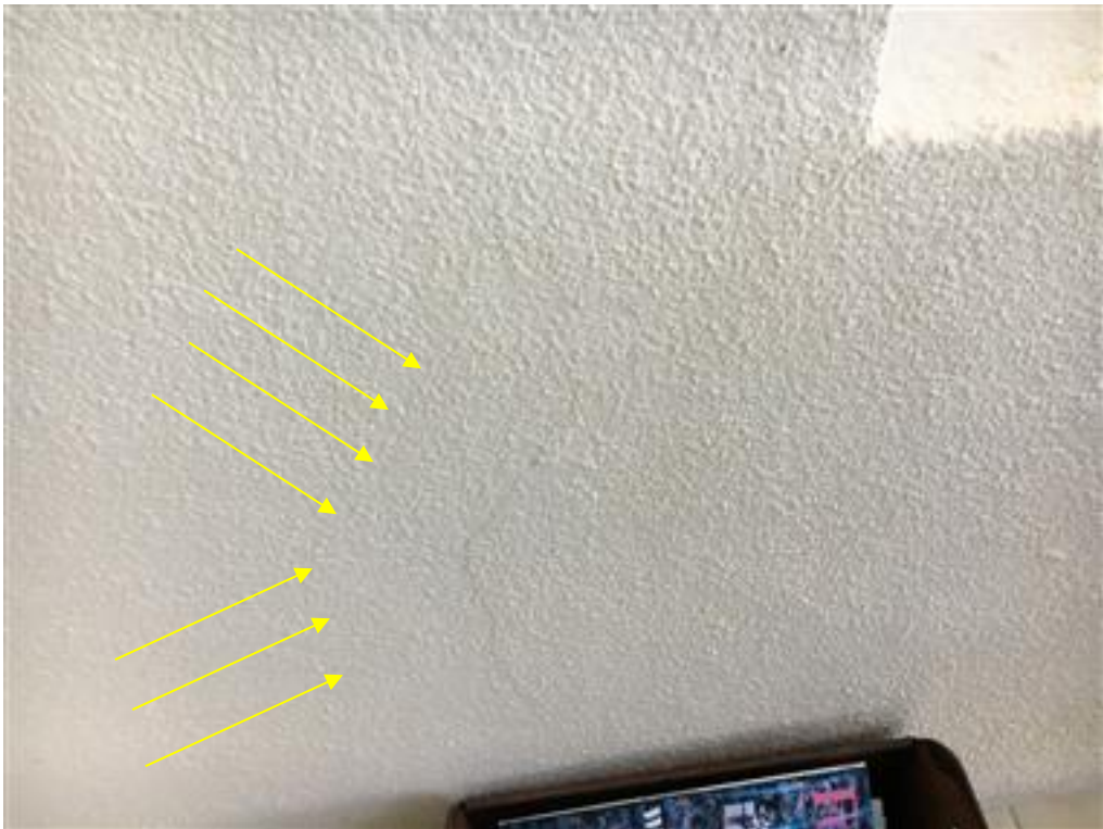
Photo 145-Unit 405, hairline crack
