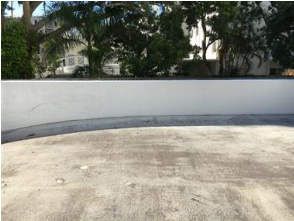
Photo 8-UPPER LEVEL WALLS- TYPICAL
