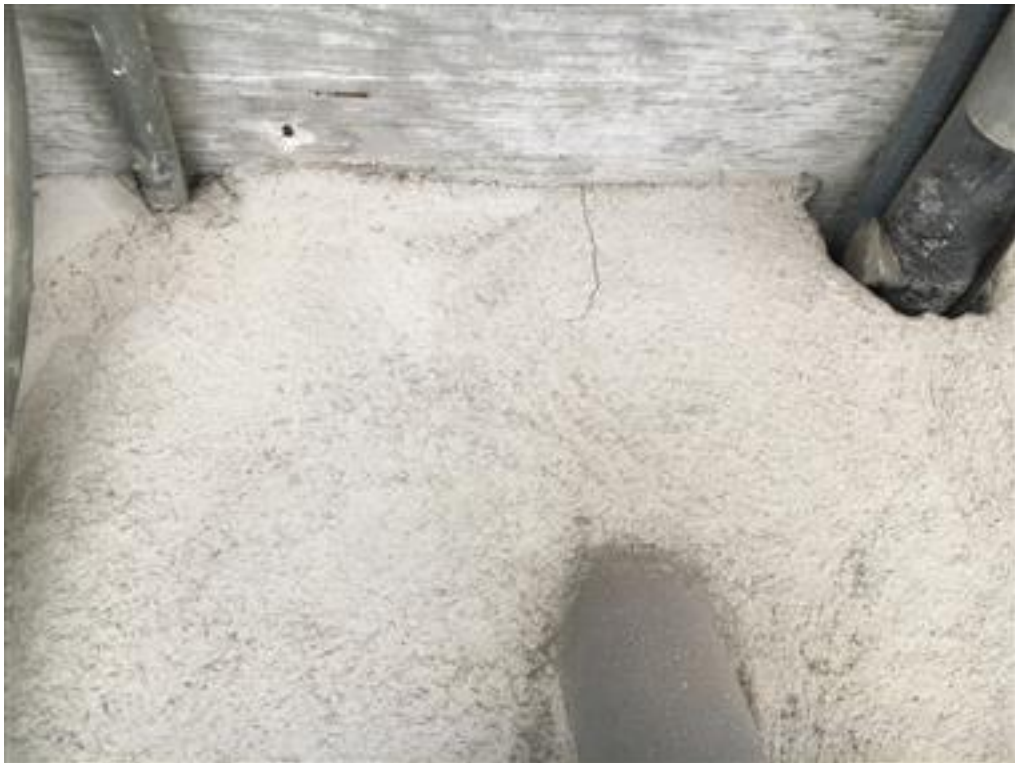
Photo 16-9 th FLOOR- HLC
