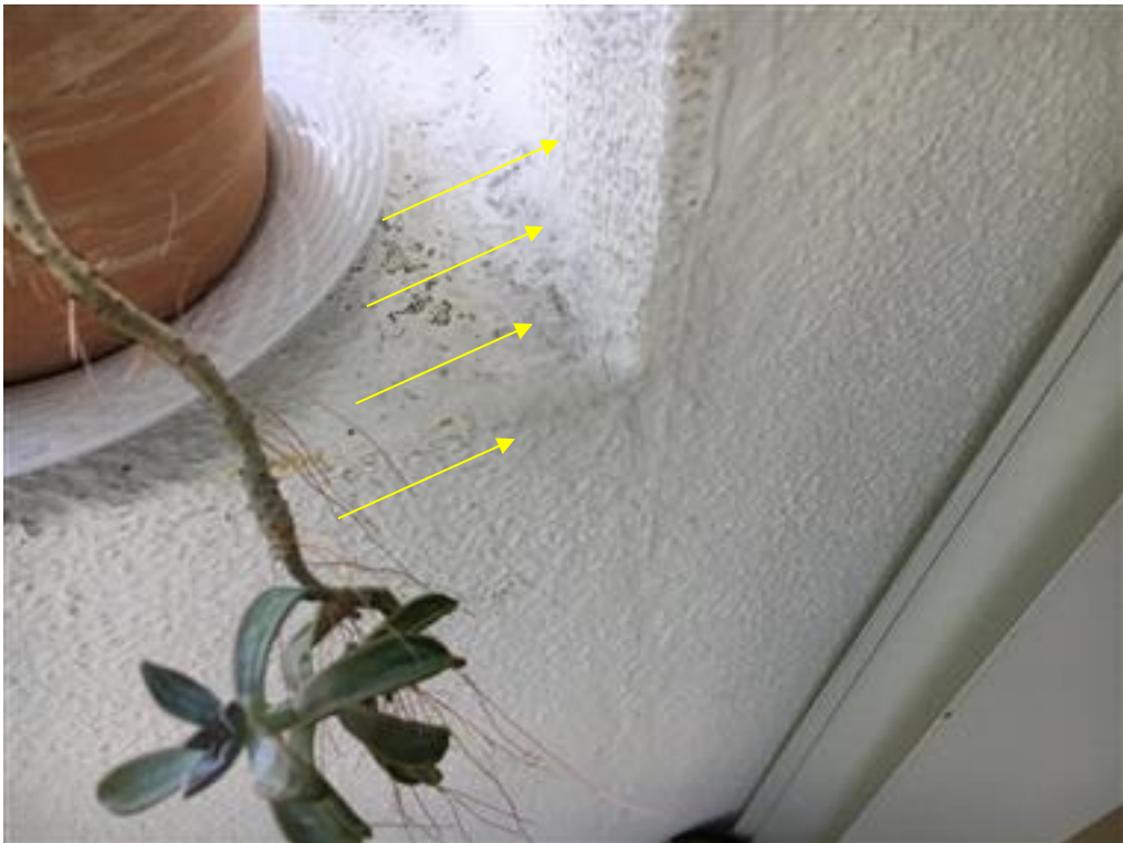
Photo 133-Unit 501, previous hairline crack repair
