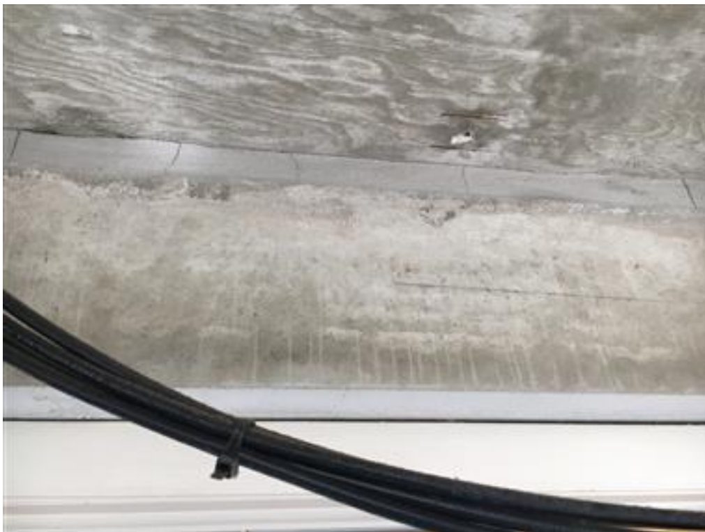
Photo 20-8 th FLOOR- HLC
