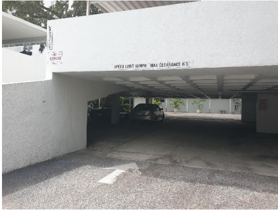
Photo 1: Overall View of Parking Garage
