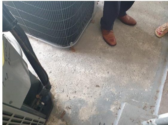
Photo 9: Condition of the slab under the MEP
