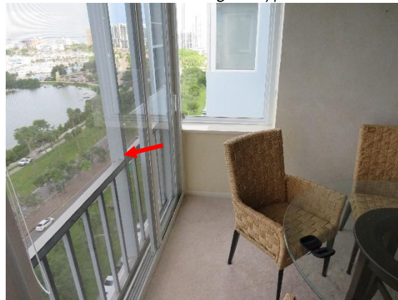
Interior Photo of Screen Enclosure Framing
