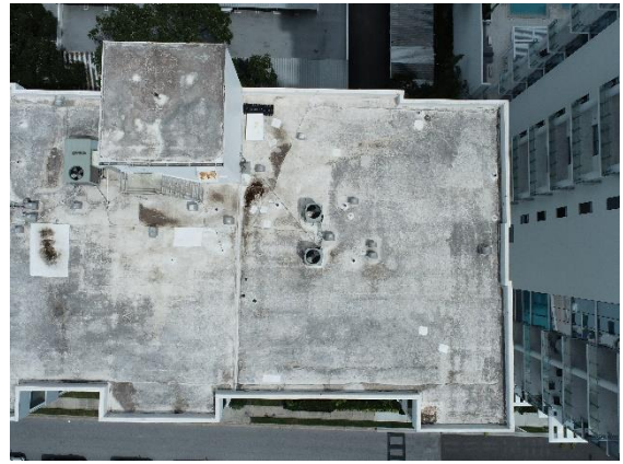
Roof Overall Photo
