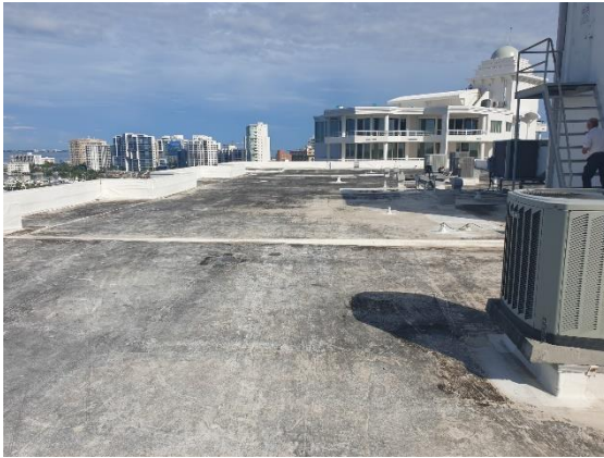
Roof Overall Photo
