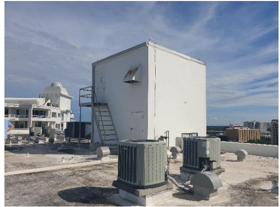
Roof Overall Photo
