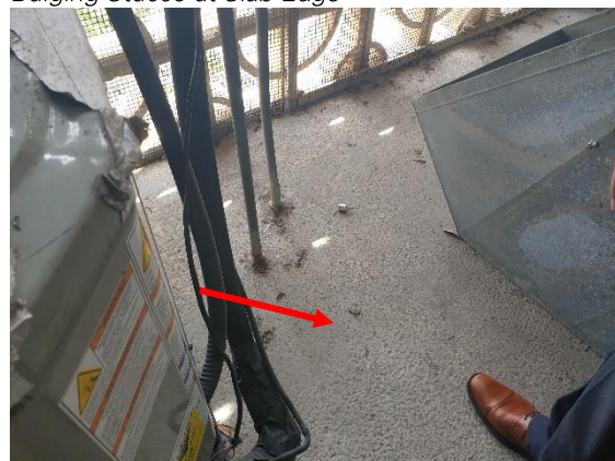
AC Condenser Area Slab
