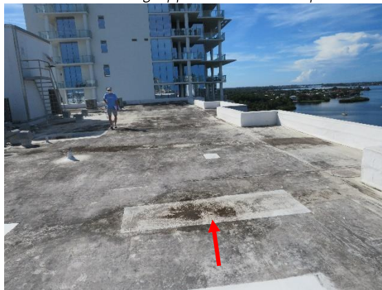
Patched Area of Coating at Rooftop
