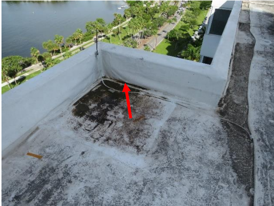
Elastomeric Coating Application at Rooftop
