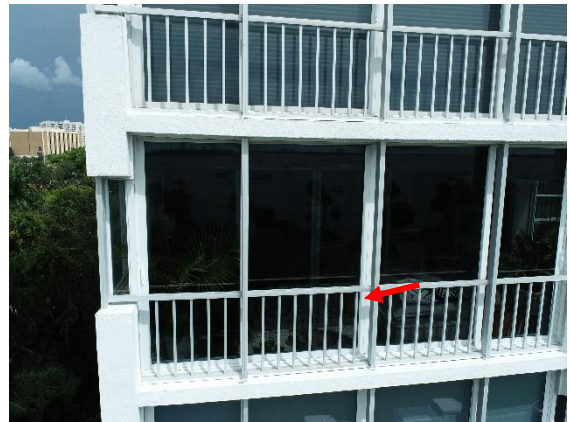
Screen Enclosure Framing at Typical Balconies
