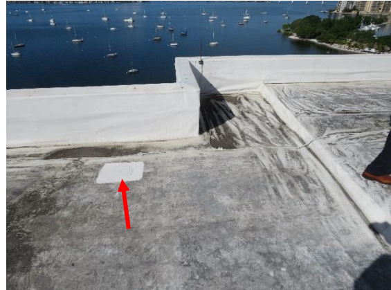
Patched Area of Coating at Rooftop
