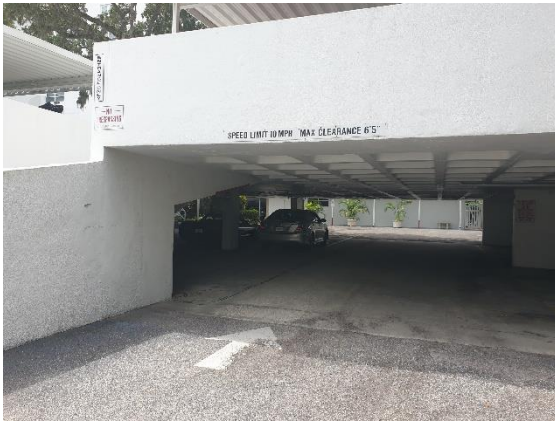
Garage Entrance Overall Photo
