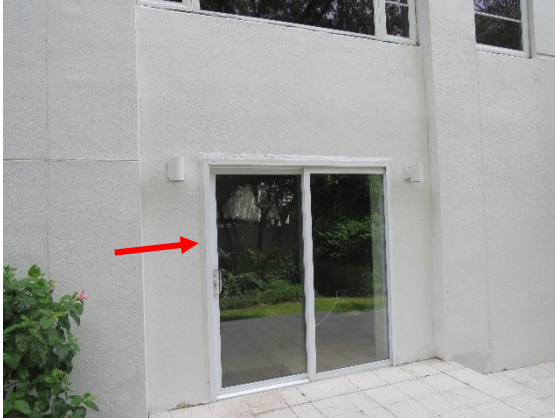
New Opening in Infill Wall
