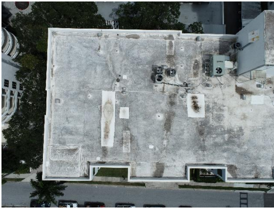
Roof Overall Photo
