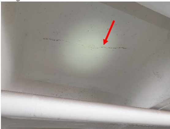
Additional Concrete Spalling
