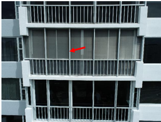
Screen Enclosure Framing at Typical Balconies
