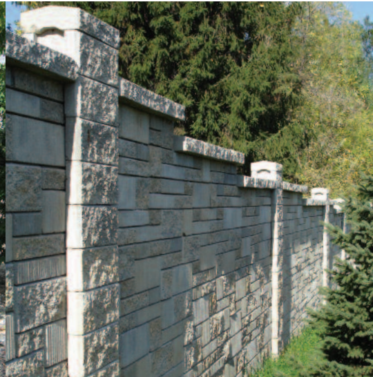
Fence / Compound Walls
