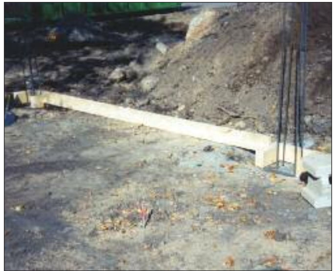
Figure 1: AB Fence Pile Layout Jig
