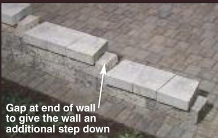
The AB Courtyard Collection is designed to let you easily step down or end the walls in a number of ways. You can also end a wall panel at a post/pillar, *see page 12 for more information.*
