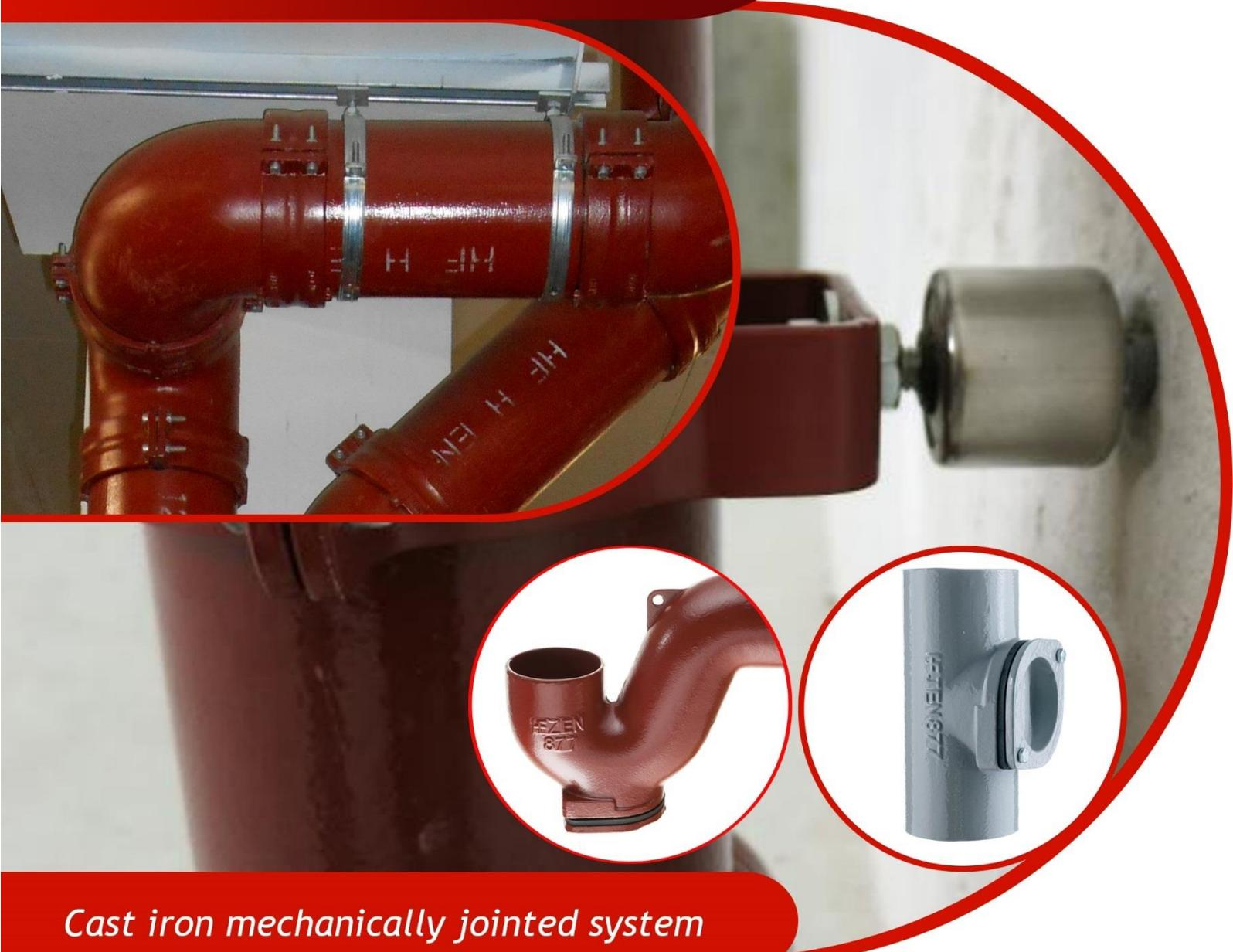
*Cast iron mechanically jointed system*
