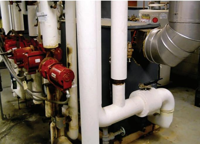
**When only one pump operated, there was insufficient flow through the boiler.**
