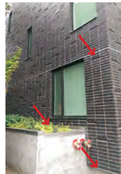
Fig. 3-16 This masonry veneer bears on continuous shelf angles (at right and above) and a concrete foundation element (at left).
