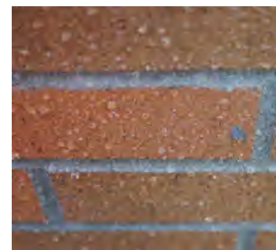
Fig. i-42 Water droplets form on a brick veneer on which clear water repellent has been applied
