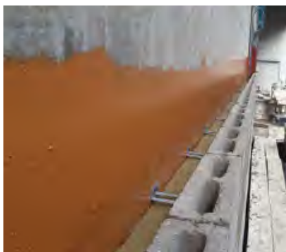
Fig. 1-5 Fluid-applied air barrier and WRB system field membrane over a concrete backup wall. Double eye and pintle masonry veneer ties penetrate through the exterior semi-rigid mineral fiber insulation.
