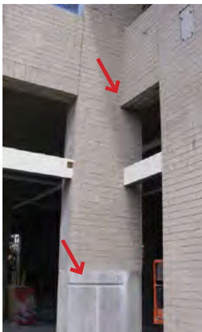
Fig. 1-20 Masonry veneer bears on concrete foundation elements below and loose lintel elements above openings as indicated
