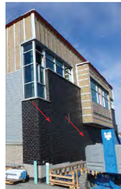
Fig. 2-20 Expansion joints (where indicated by red arrows) are located on this veneer where transitions occur at window steps and wall projections. Joints are continuous from the foundation-bearing element to the full height of the veneer.
