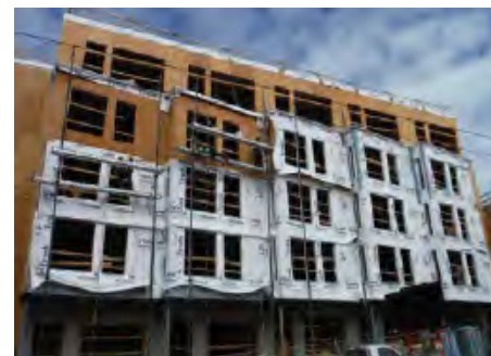
Fig. i-17 Sheet-applied air barrier and water-resistive barrier membrane example
