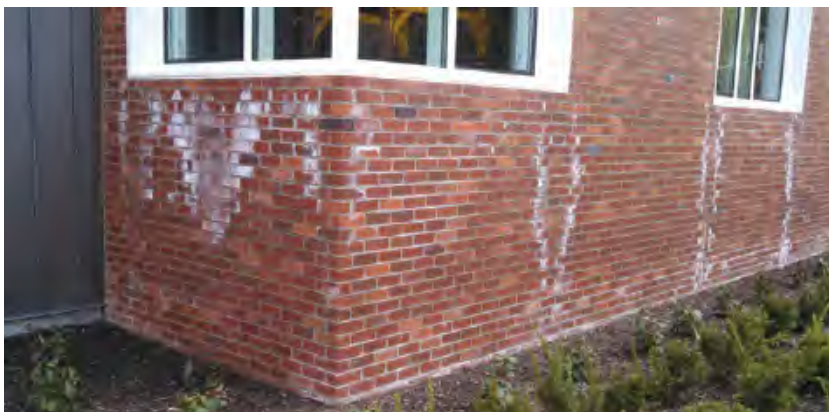
Fig. i-45 Example of efflorescence on anchored masonry veneer
