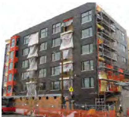
Fig. 3-2 Wood-framed wall with anchored masonry veneer example project application
