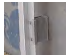
Fig. 8-9 Cladding support clip options including an intermittent Z-girt (top) and fiberglass standoff clip (bottom)
