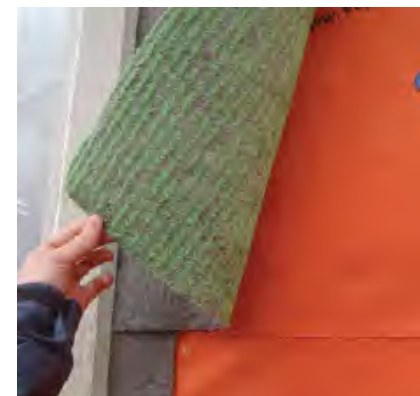
Fig. 8-10 Drainage matrix over a mechanically fastened air barrier and WRB system field membrane with sealed laps.
