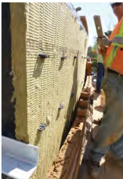
Fig. 2-5 Semi-rigid mineral fiber insulation with thermally optimized masonry ties
