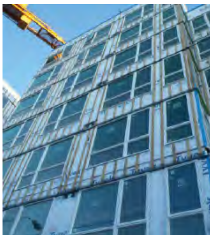
Fig. 8-4 Furring strips secure the sheet-applied air barrier and WRB system
