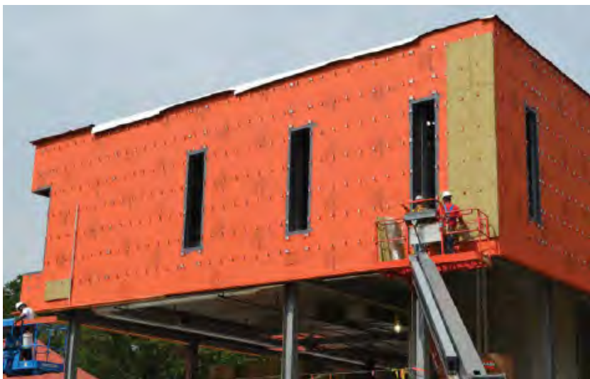
Fig. 7-4 Self-adhered sheet air barrier and WRB field membrane with fluid-applied flashings at rough openings and exterior semi-rigid mineral fiber insulation
