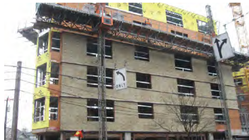
Fig. i-20 Semi-rigid mineral fiber insulation prior to anchored masonry veneer installation
