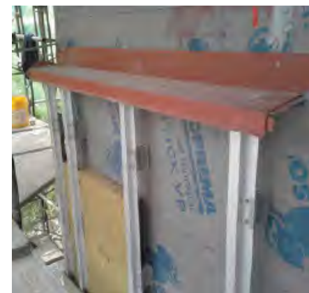
Fig. 7-12 Fiberglass clip with continuous Z-girt, semi-rigid insulation, and prefinished cross-cavity sheet-metal flashing
