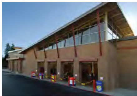
Fig. 4-2 CMU wall with integral insulation example project application
