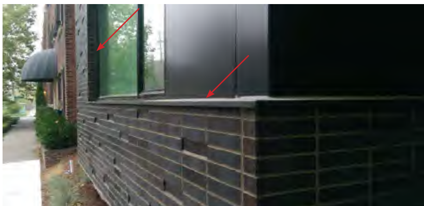
Fig. 2-19 A sheet-metal flashing conceals the top of the rainscreen air cavity and masonry at this windowsill area. The sheet-metal flashing extends beyond the masonry veneer face to deflect water away from the veneer. At the window jamb condition beyond, sheet-metal trim is also used to close off the rainscreen air cavity.
