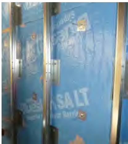
Fig. 7-13 Intermittent Z-girt cladding support clips and continuous Z-girts. Mechanical impaling pins are attached between framing members for additional support of the exterior insulation. Note that a Class I (vapor permeance) air barrier and WRB system is depicted in this figure, which is typically acceptable where cavity insulation is minimized to 1/2 to 1/3 of the total nominal insulation R-value of this system and vapor control layer at the interior side of the framing is eliminated.
