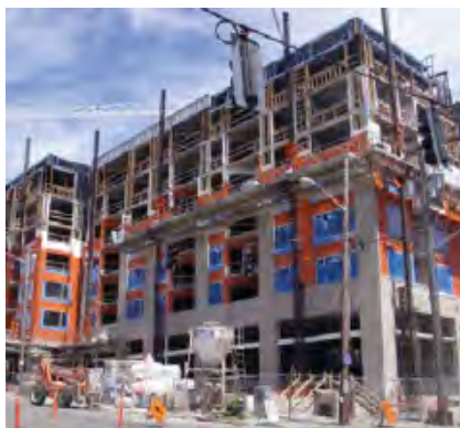
Fig. 2-2 Steel-framed wall with anchored masonry veneer example project application
