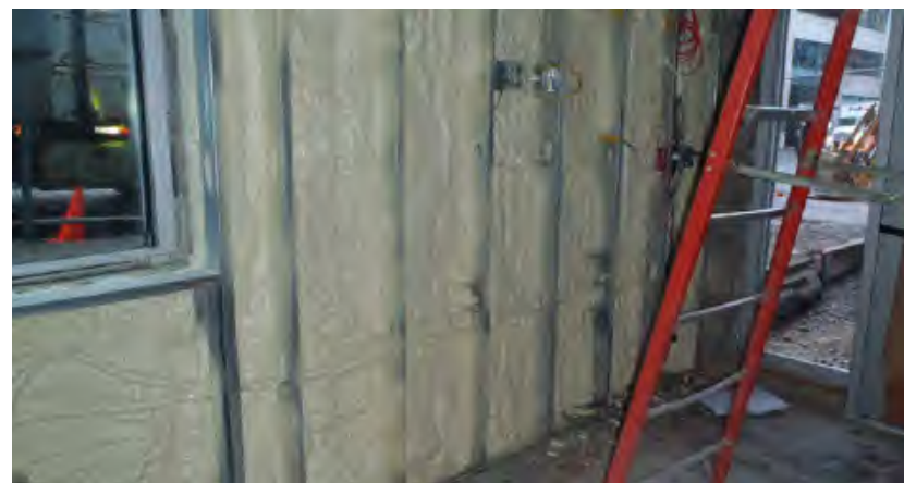
Fig. 5-4 Closed-cell spray foam insulation installed between steel studs
