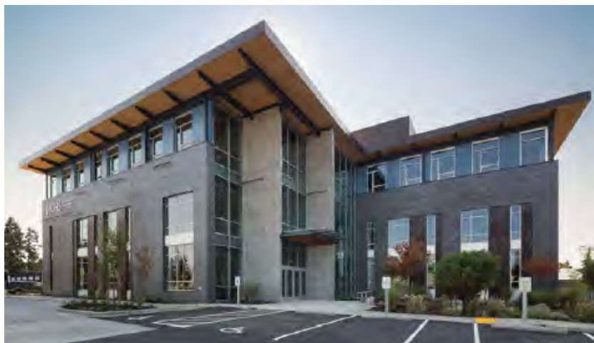
Fig. i-10 ICHS Shoreline Medical and Dental Clinic, constructed in 2014, features large roof overhangs and canopies above entrances to deflect rain away from the above-grade enclosure components and shade the interior environment from the sun.
