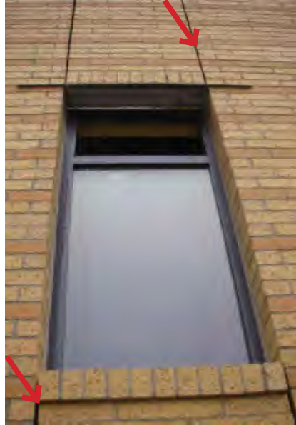
Fig. 1-18 Typical vertical brick expansion joint aligned with window jambs. Each joint continues the full height of the building and is awaiting backer rod and sealant joint installation.
