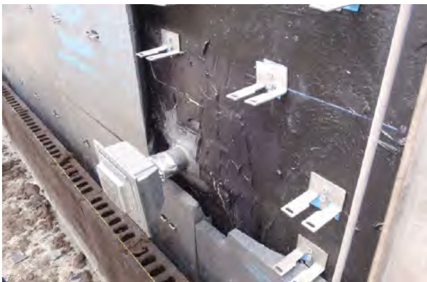
Fig. 2-4 Double eye and pintle plate ties are attached through self-adhered membrane patches over top of the fluid-applied air barrier and WRB systems. Ties penetrate the continuous rigid insulation.
