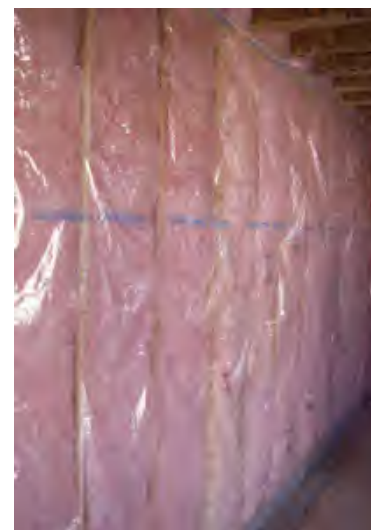
Fig. i-19 Polyamide film vapor retarder installed over a wood-framed wall with cavity batt insulation
