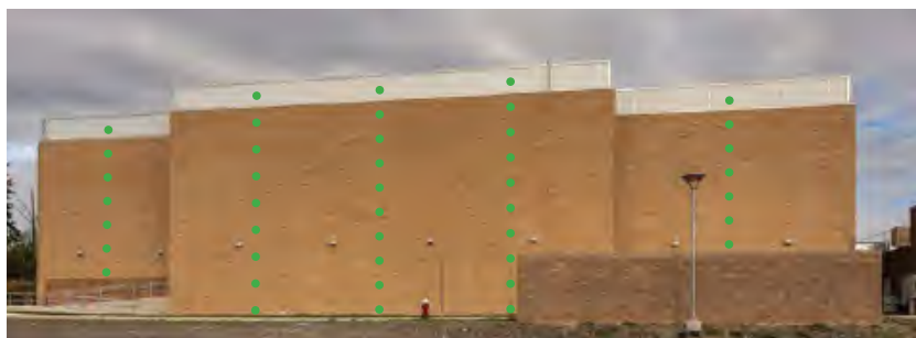
Fig. i-33 Example of vertical CMU control joint locations (shown in green)
