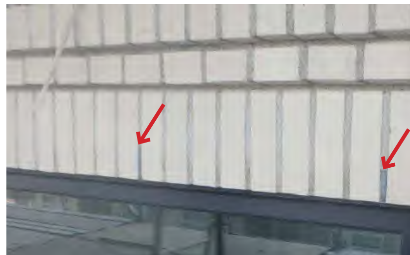
Fig. 3-14 Mesh weep/vents located within the head joints of a soldier course of lip brick. The base of each weep/vent is tight to an underlying cross-cavity sheet-metal flashing, which is concealed by the lip brick.
