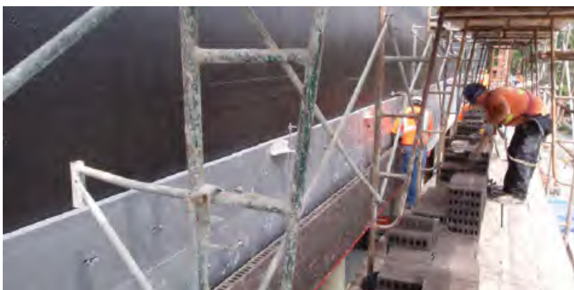
Fig. i-21 XPS insulation behind anchored masonry veneer
