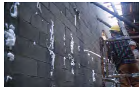
Fig. 4-4 Installation of foam-in-place CMU core insulation
