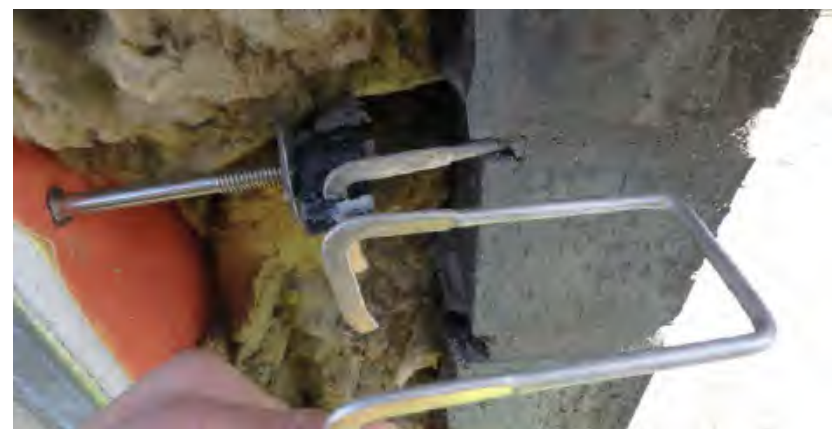
Fig. 1-21 Thermally optimized screw tie with stainless-steel hook and barrel as observed at a freestanding mock-up
