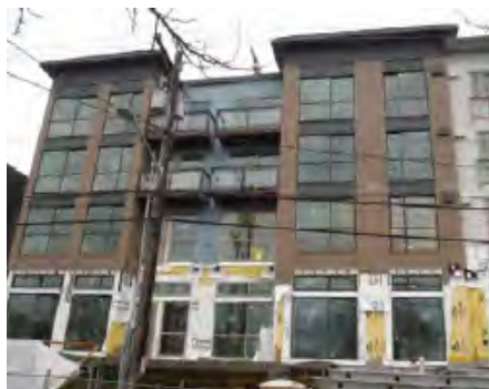
Fig. 7-2 Steel-framed wall with adhered veneer example project application
