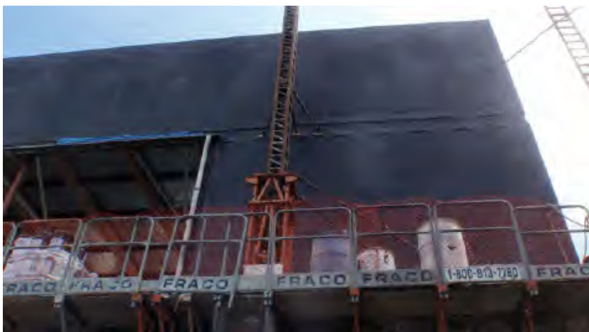
Fig. 6-4 Fluid-applied air barrier and WRB field membrane installed over CMU wall substrate
