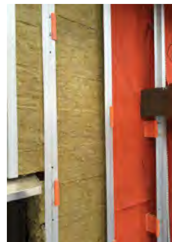
Fig. 8-6 System 8 Option B on intermittent cladding support clips. Refer to Chapter 7 for exterior insulation selection and cladding attachment discussion.
