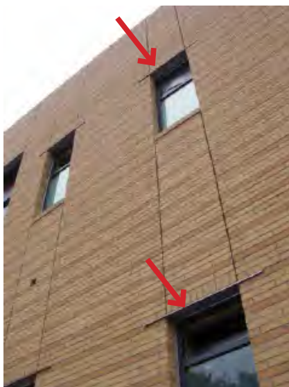
Fig. 2-22 Loose lintel supports (with a sheet-metal flashing) occur at small window head conditions on this elevation.
