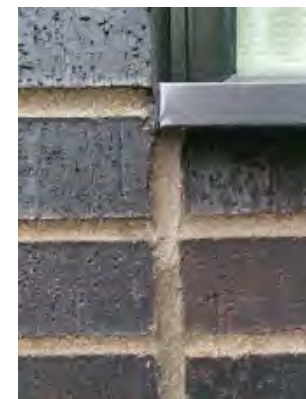
Fig. i-35 Typical sanded sealant joint below a window opening
