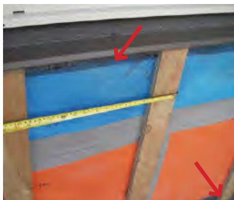
Fig. 8-13 Preservative-treated furring strips over a mechanically fastened air barrier and WRB system field membrane. Insect screen wraps around the top and bottom of the furring strips to close off the air cavity from insects while still allowing for drainage and ventilation.
