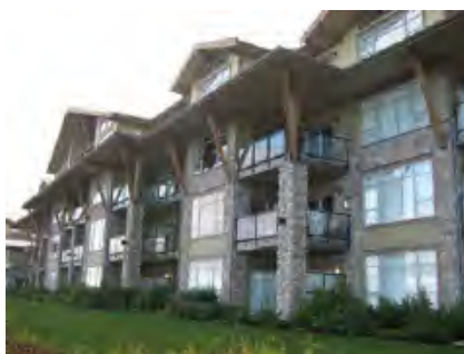
Fig. 8-2 Wood-framed wall with adhered veneer example project application
