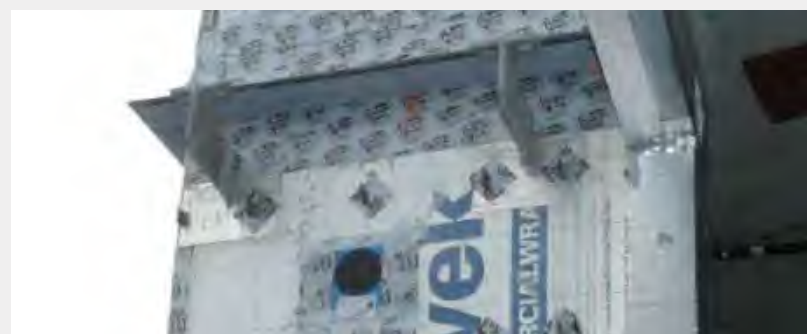
Fig. i-39 Typical structural knife plate penetrations flashed with a foil-faced self-adhered flashing membrane similar to the sequence in Fig. i-40 on page i-57. Also visible is a pre-formed penetration boot for a pipe penetration.
