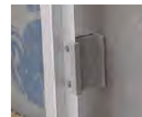
Fig. 7-7 Cladding support clip options including intermittent Z-girt (top) and fiberglass standoff clip (bottom)
