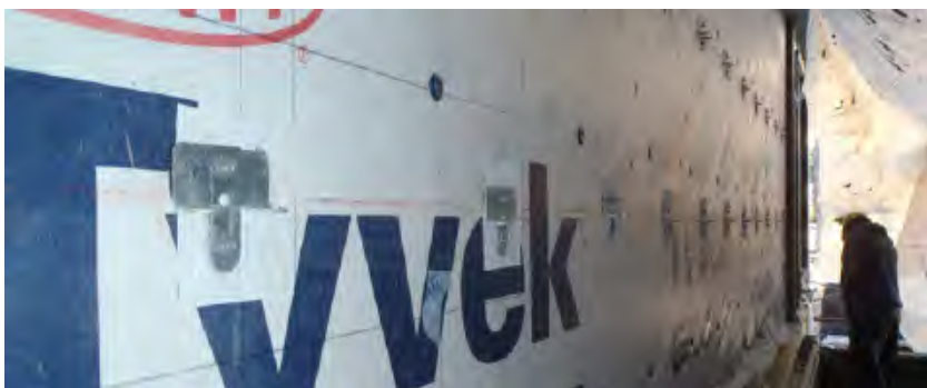
Fig. 3-4 Double eye and pintle plate ties are fastened through compatible self-adhered membrane patches over a mechanically attached sheet air and water barrier membrane.
