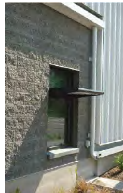
Fig. i-11 (above) Baker Middle School (opened in 2012) showcases roof overhangs that assist in deflecting rainwater away from the building enclosure below. Sun shades over windows also assist with controlling solar loads and reducing rain exposure.
