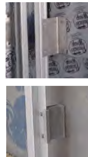
Fig. 6-5 Cladding support clip options including intermittent Z-girt (top) and fiberglass standoff clip (bottom)
