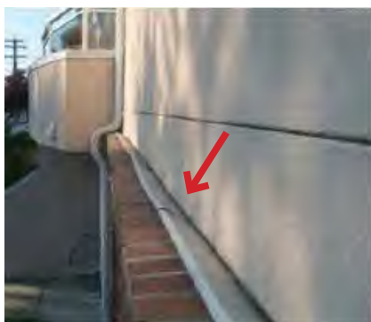
Fig. i-32 Cross-cavity sheet-metal flashing displacement as a result of wood-framed wall shrinkage and brick anchored clay masonry veneer expansion
