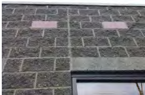
Fig. 4-5 Vertical CMU control joint
