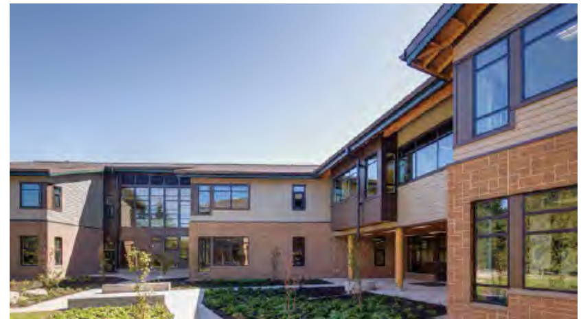
Fig. i-5 Many building enclosure elements are visible in this photo, including a roof, above-grade walls, windows, doors, and floors (i.e., soffits).
