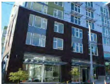
Fig. 6-2 Adhered CMU wall with adhered veneer example project application
