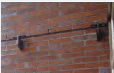
Fig. i-38 Typical structural knife plate penetrations through an anchored masonry veneer prior to installation of exterior sealant joints or final cleaning
