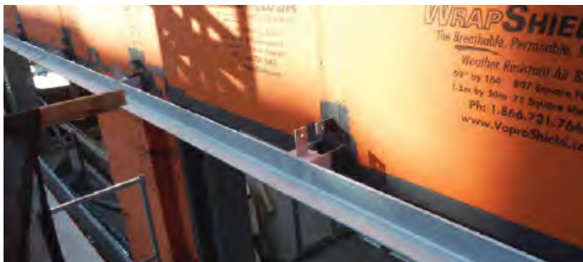
Fig. 1-8 Hot-dipped galvanized standoff shelf angle
