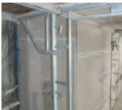
Fig. 7-14 Cement backer board installed over exterior insulation and cladding support system
