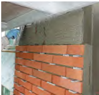
Fig. 7-16 In-progress installation of masonry veneer over thinset mortar and crack isolation membrane
