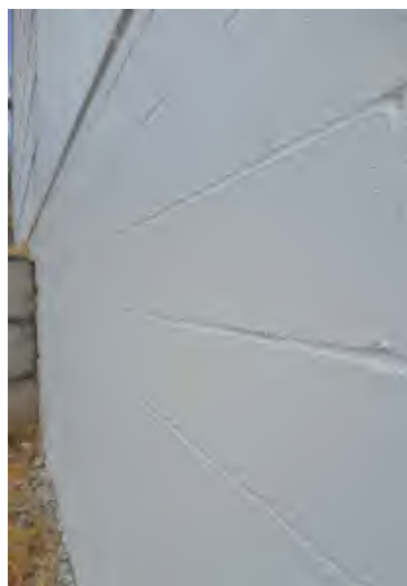
Fig. i-44 Exposed CMU wall coated with elastomeric coating
