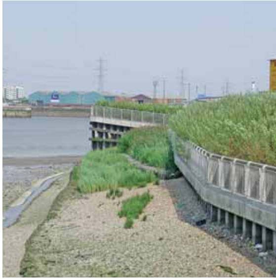
Intertidal terraces and environmental signage at the Greenwich Peninsula, London
