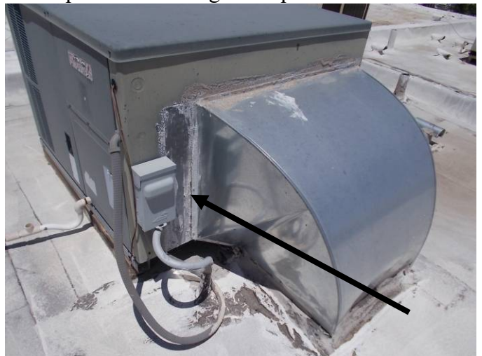
The seal at the duct work/HVAC unit joint is not sealed in a watertight manner.
