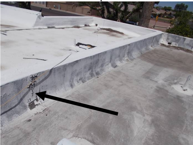
The wall flashing lapped are cracked apart. The aluminum coating has completely deteriorated.
