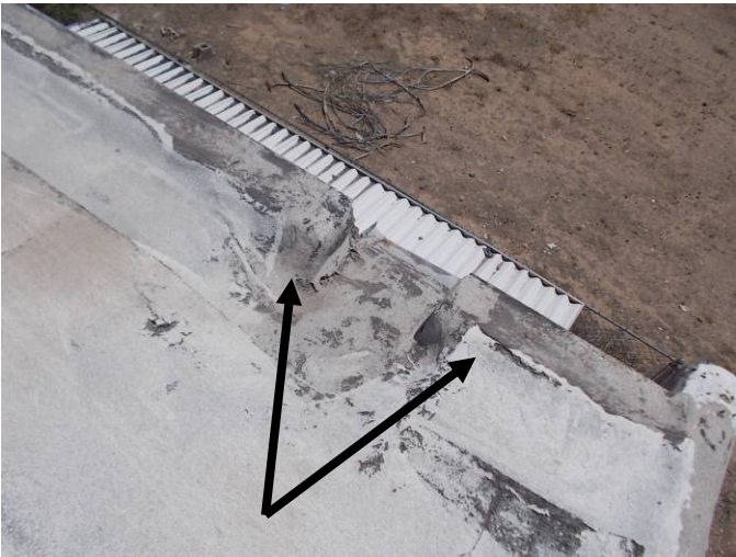
The seal around the scupper is not watertight. The wall flashing is splitting apart.
