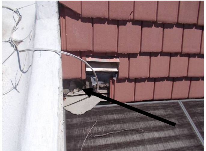
The area around the outside of the scupper on the tile mansard is not watertight. Decking is exposed.
