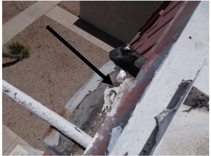
The seal around the scupper at the BUR system and the tile mansard are not watertight.
