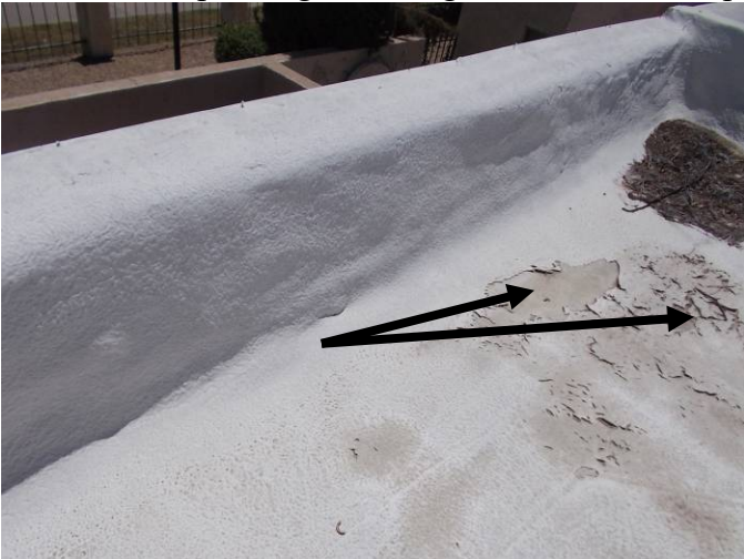
The coating has peeled up and is deteriorated which is accelerating the deterioration of the roof system.
