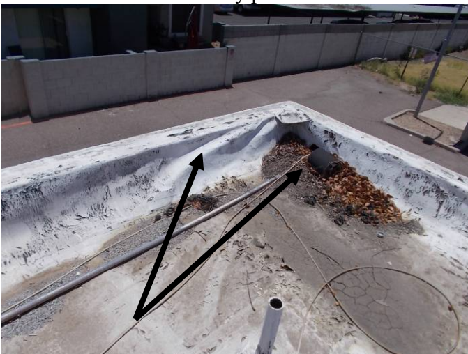
The PVC line is run through the scupper contributing to the debris build up which is impeding proper drainage. Wall flashing buckled.
