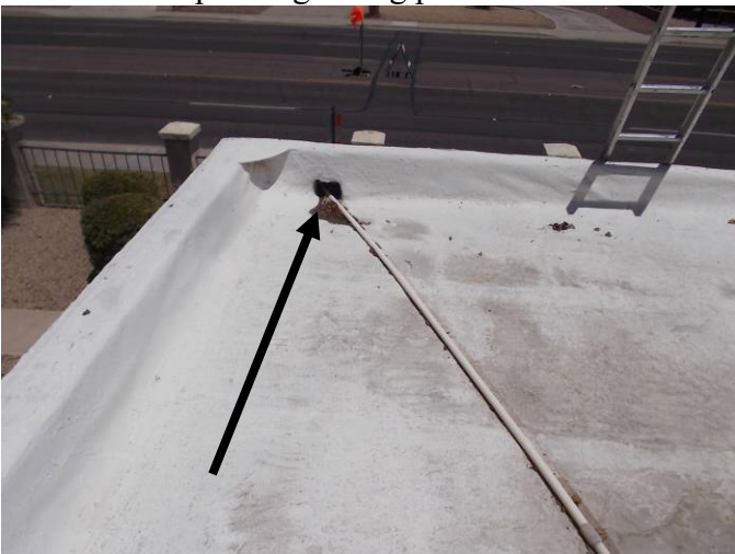
The PVC line has been run through the scupper which impedes the flow of water off the roof and promotes debris build up in front of the scupper.
