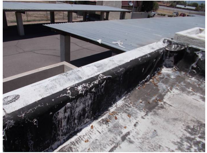
The coating on this BUR roof system has completely deteriorated.
