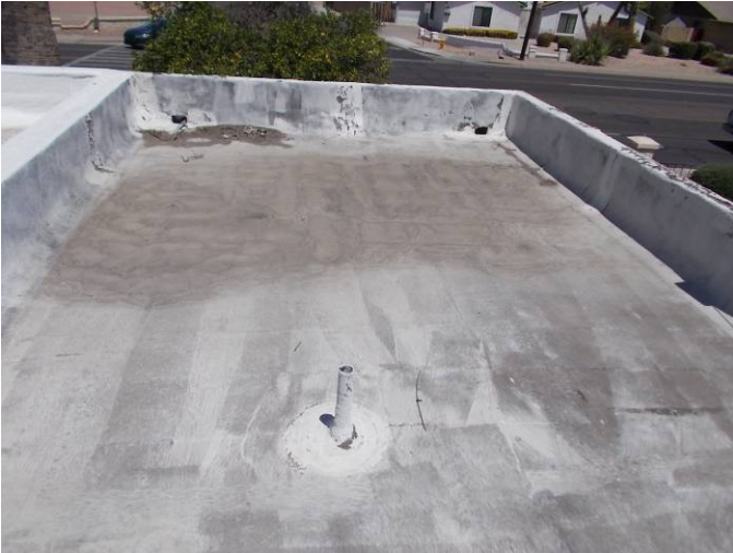
This is an overview of a single BUR system on 8405 N. 59 th Drive. It is in poor condition.
