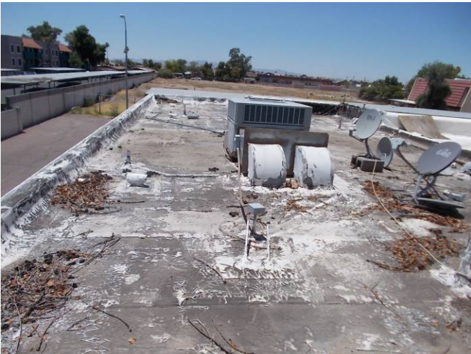
This is an overview of the BUR roof system at 8315 N. 59 th Dr. which is in very poor condition.
