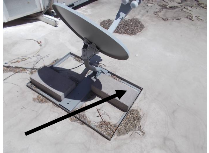
The TV dish mounting stand does not have a protective slip sheet under it which poses a puncture risk to the system.
