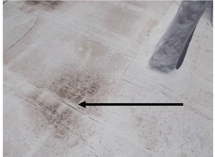
The roofing membrane has split open and is allowing water penetration.
