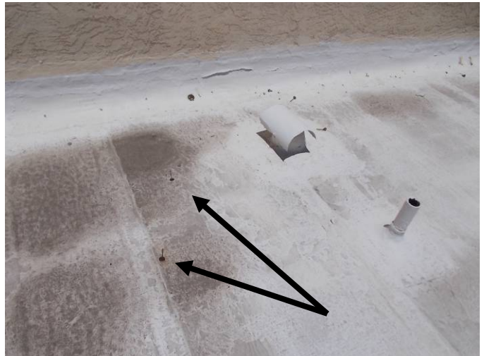
These are fasteners from previous work on the building that have been left on the roof and pose a puncture hazard to the roof system.
