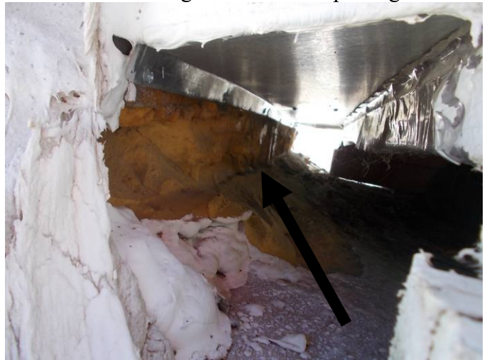
Underneath the HVAC unit at the duct work is not coated and not sealed in a watertight manner.
