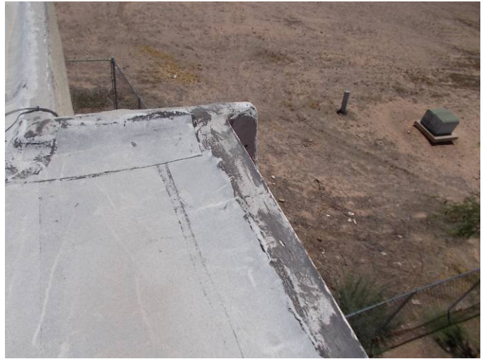
The top of the wall flashing is coming apart and susceptible to water penetration.
