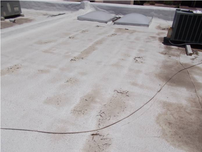
This is an overview of the foam roof system on 8331 N. 59 th Dr. which is in very poor condition. The coating is cracking, peeling, & splitting. The coating is severely deteriorated.
