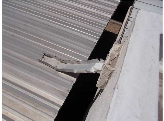
A make shift scupper extension has been installed on the west end. The exterior stucco pop-out is cracked open and susceptible to water penetration.
