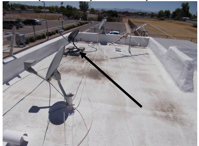
There is an excessive amount of TV dishes on this deck and there is no protective slip sheets used.
