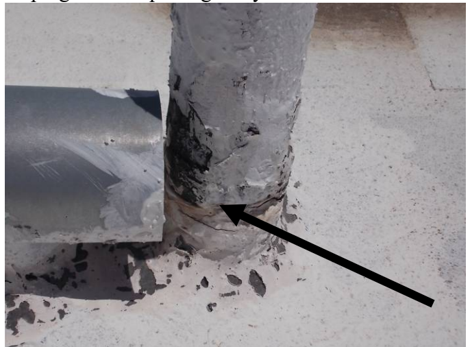
The seal around the pipe roof penetration is not watertight.
