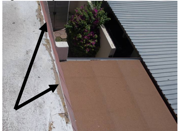
The roof has deteriorated along the metal edge and is allowing water penetration.
