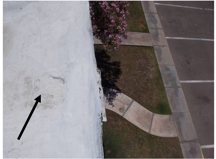
There are splits in the coating and roof system in front of the scupper.
