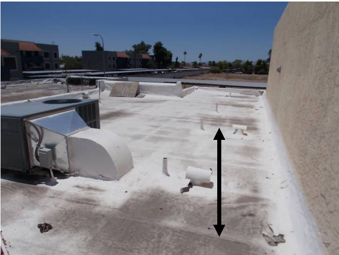
This is an overview of the BUR roof system on 8319 N. 59 th Dr. which is in fair condition. Considerable ponding taking place
