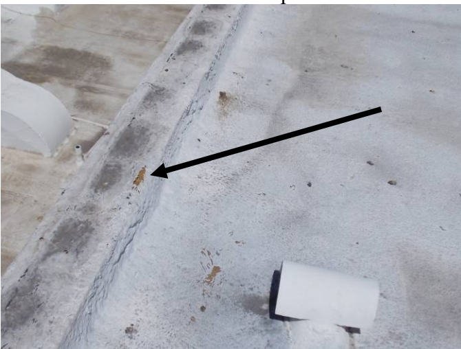
The coating is deteriorated to the point where the foam is exposed to UV rays which will accelerate the deterioration of the roof system.
