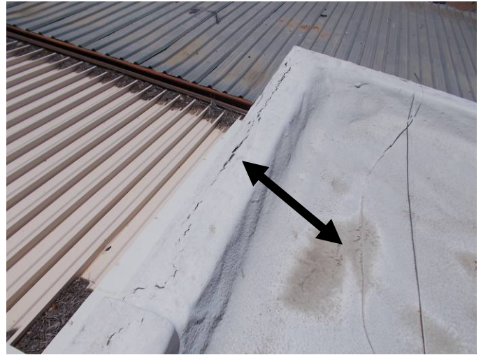
The top of the wall flashings are cracking and pulling apart. Cracking in deck coating.
