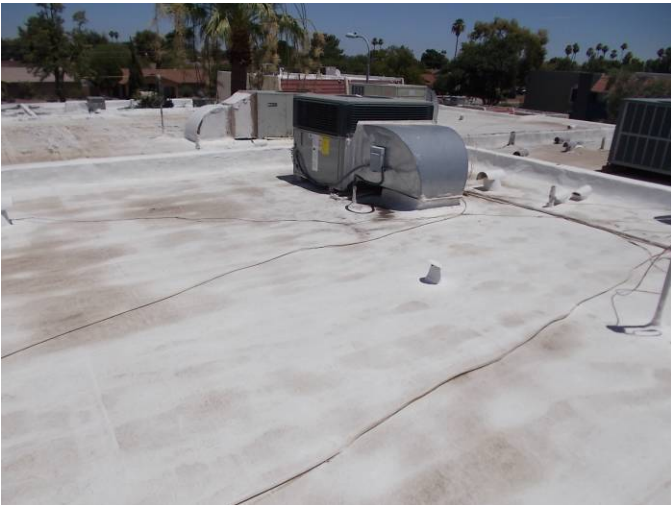
This is an overview of the BUR system on 8340 N. 59 th Dr. The roof is in poor condition.
