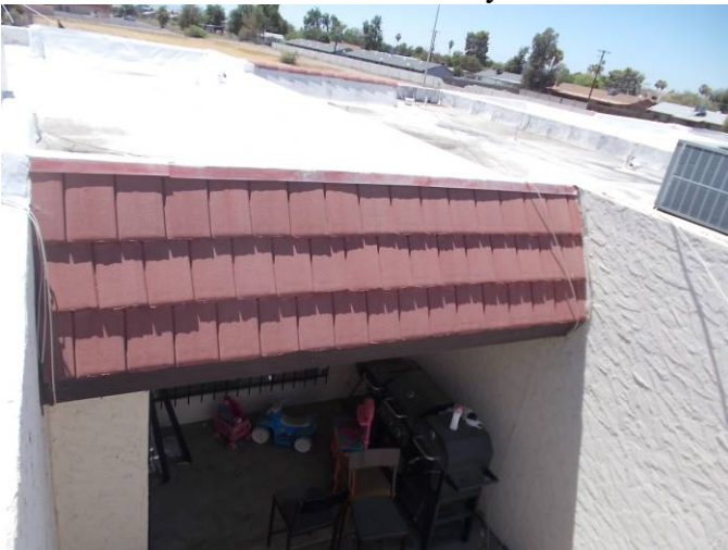
This is a view of the tile mansard which has no scuppers coming through it.
