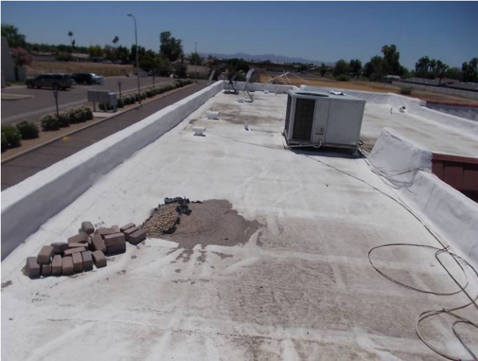
This is an overview of the BUR system on 8401 N. 59 th Drive which is in poor condition. Large amounts of debris on roof. 3 roof systems exist.
