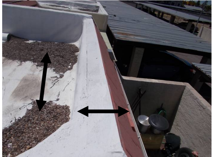
Excessive debris on this deck. Dormant scupper seen on tile mansard none on BUR deck.
