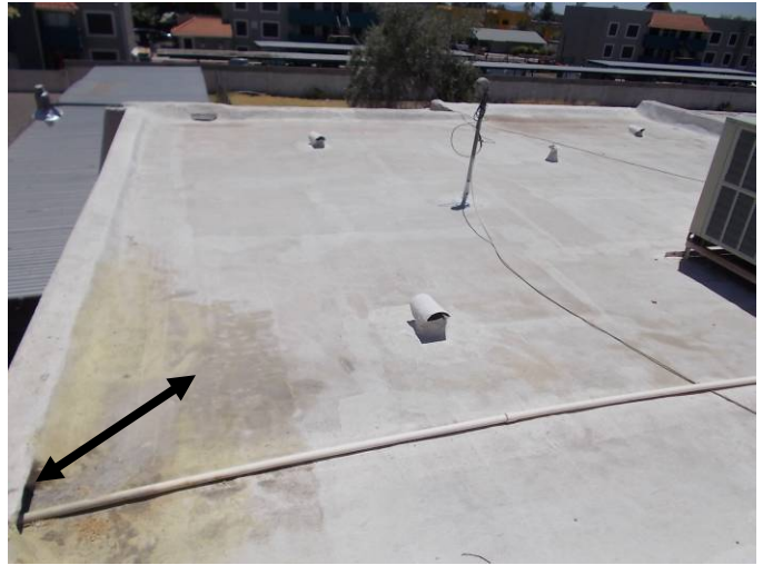
The coating is deteriorated due to ponding water near the parapet wall and scupper. The PVC through the scupper is impeding water flow.
