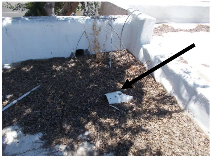
The debris has completely covered a t-top and water is not draining properly off the roof. Coating deterioration is accelerated.
