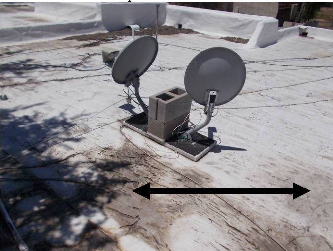
This area which ponds water has deteriorated coating which is no longer protecting the roofing membrane below it.
