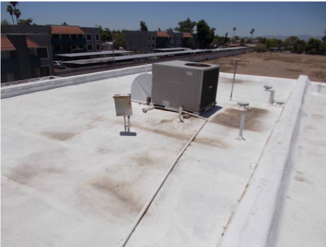
This is an overview of the BUR system which is in fair to poor condition on 8323 N. 59 th Dr.
