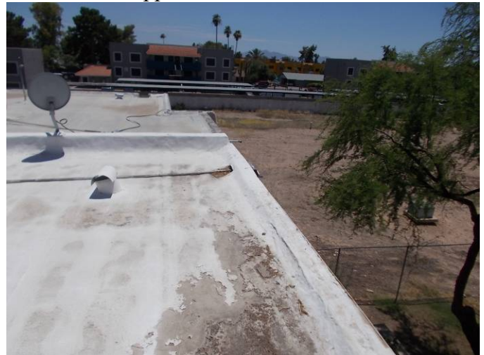
The coating has peeled away and deteriorated due to ponding water. The PVC line is run through the scupper and is impeding water flow.
