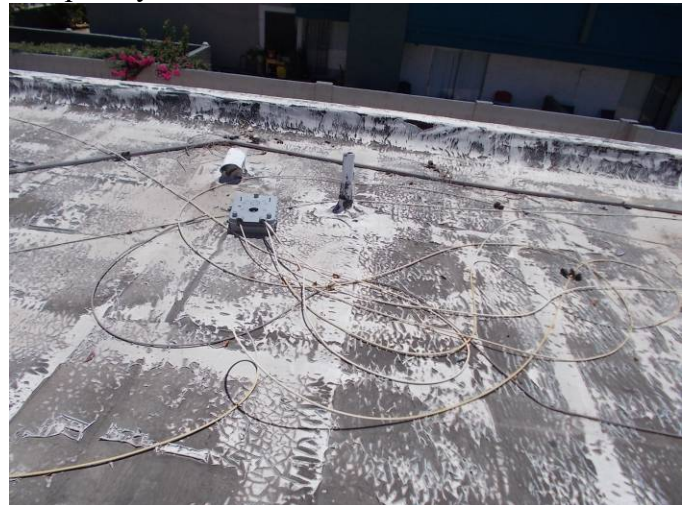
Numerous cracks and splits in the roofing membrane were found. Lots of debris on roof
