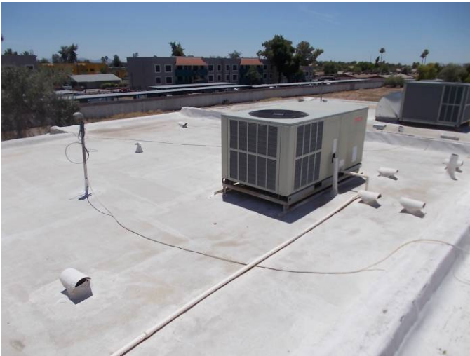
This is an overview of the BUR system on 8328 N. 59 th Drive. It is in fair to poor condition.
