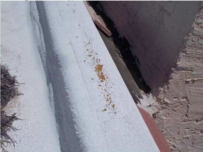
The foam below the coating is exposed to the UV rays which will decrease the life of the roof.
