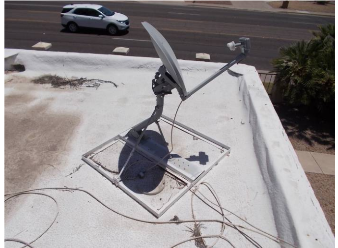
There are numerous areas which pond water on this deck. The TV dish mounting platform does not have a protective slip sheet under it posing a puncture risk to the roof system.
