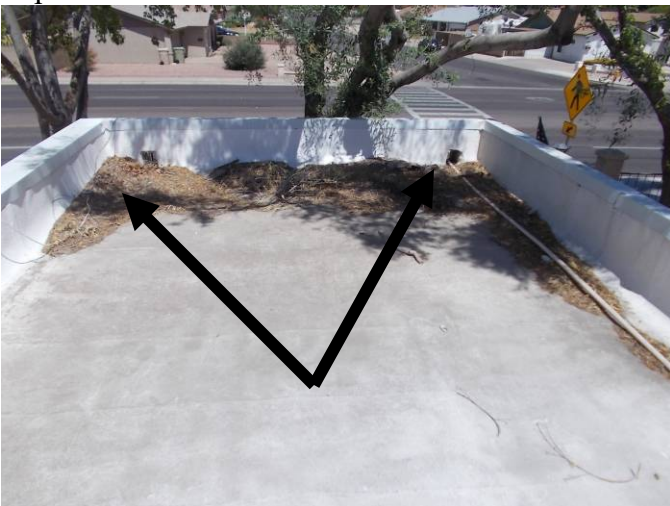
Large amount of debris on the roof deck. PVC line running through scupper which is promoting debris build up and is impeding water flow off roof.
