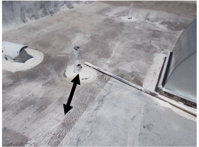
There is a hole in the side of the pipe penetration and is allowing water to leak. Roofing membrane coating is alligatoring.
