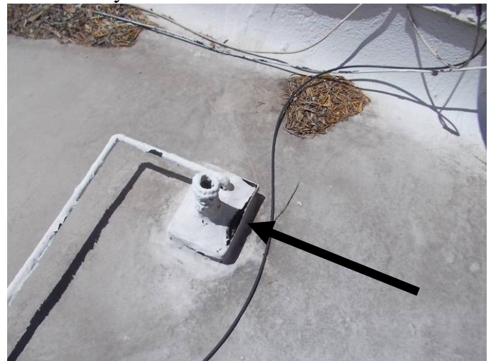
The pitch pan is not in a watertight condition and is susceptible to water penetration.
