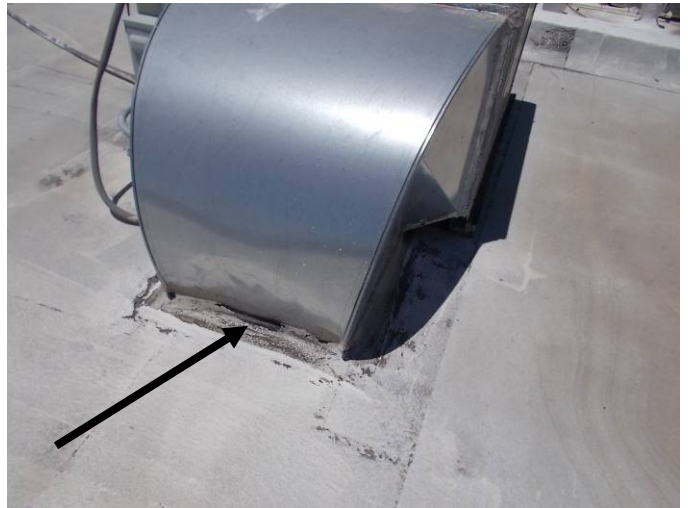
The seal around the base of the HVAC duct work is wide open and allowing water penetration.
