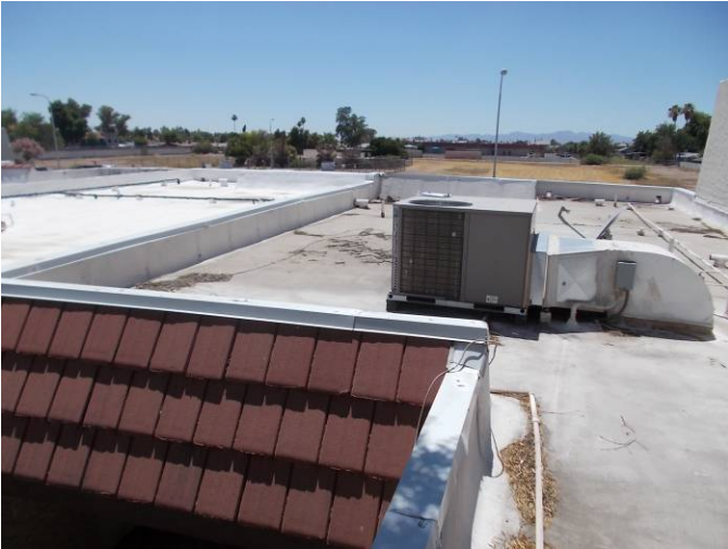
This is an overview of the tile mansard roof and the BUR system on the low-slope deck which is in fair to poor condition.
