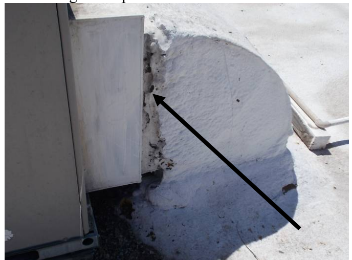
The joint between the duct and the HVAC unit is not sealed in a watertight condition and is allowing water to penetrate.
