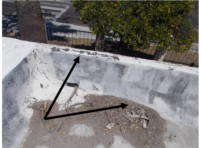
Water is ponding in area of scupper and debris is built up as well. Top of wall flashings failing.
