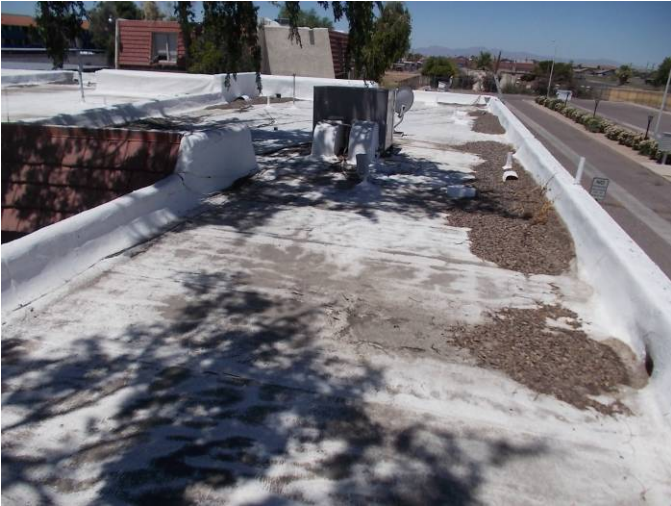
This is an overview of the BUR system on 8343 N. 59 th Dr. which is in poor condition.
