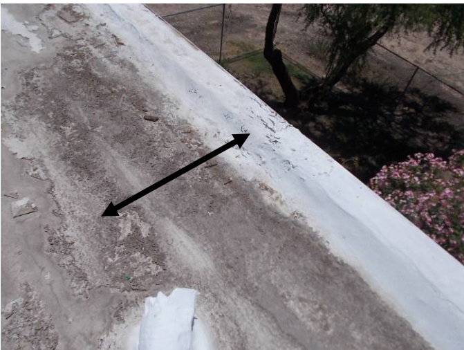
Ponding and coating deterioration occurring along this section of parapet wall. Cracking in top of wall.
