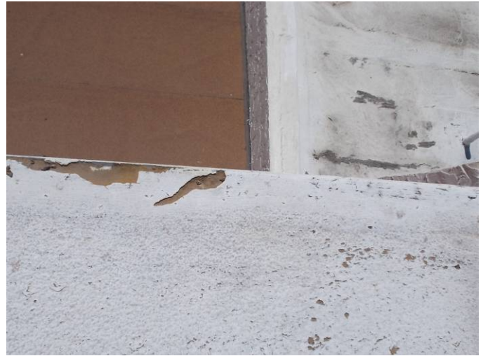
The foam is exposed and cracked along the metal edge and susceptible to water penetration.
