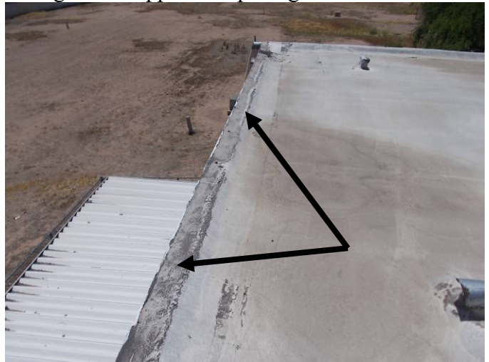
The coating at the top of the wall flashings have deteriorated and the seal along the wall is splitting.
