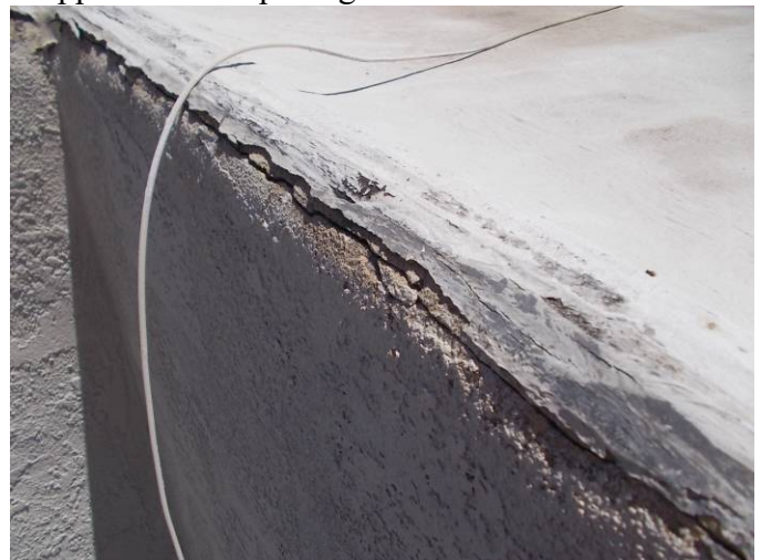
The top of the parapet wall on the north side is cracked wide open and allowing water penetration.
