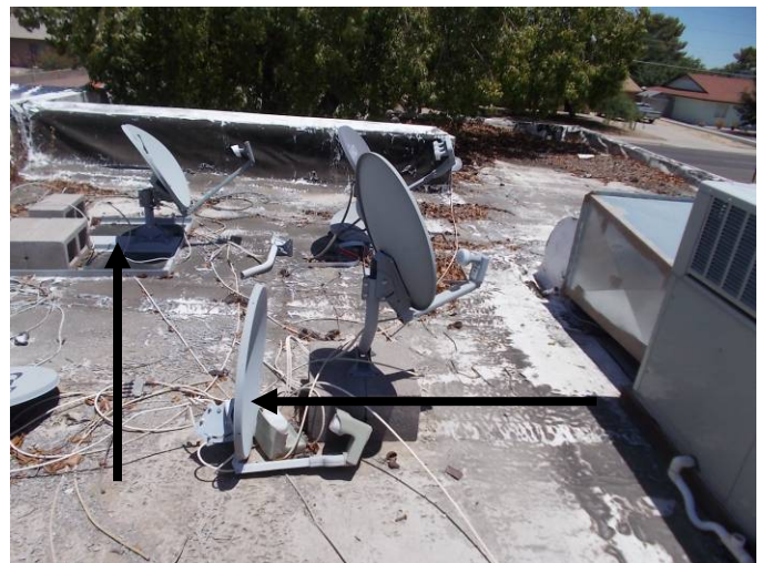
There are abandon TV dishes on this roof which present a puncture hazard to the roofing membrane. The dish mounts don't have slip sheets under them.
