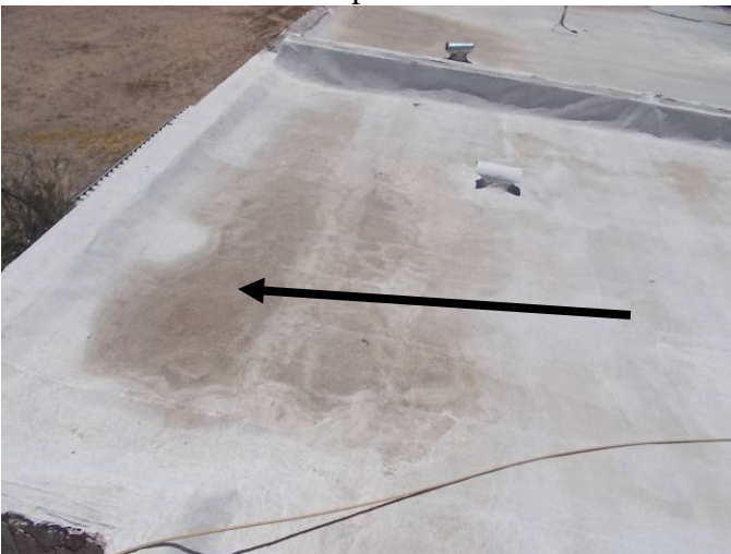
Water is ponding on this roof system which has deteriorated the elastomeric coating.
