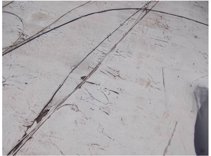
Numerous cracking and splitting of the coating and the roofing membranes which is susceptible to water penetration.
