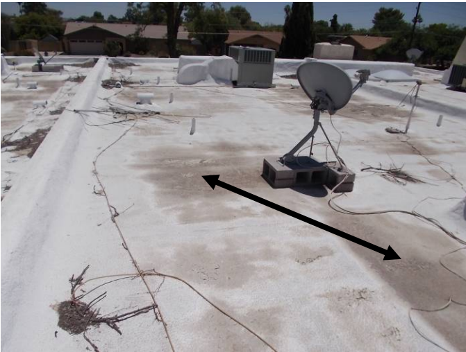
This is an overview of the foam roof system on 8335 N. 59 th Dr. which is in poor condition. Considerable ponding occurring and debris build up
