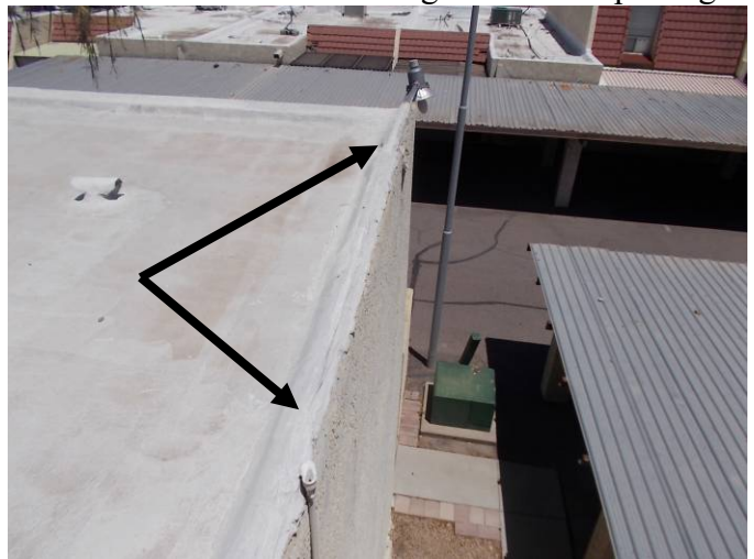
It is unacceptable to have the street light electrical conduit encapsulated by the roofing material.
