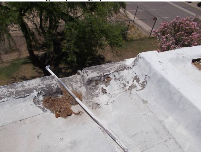
The PVC line is impeding the flow of water off the roof and contributing to debris build up and deterioration of the coating.
