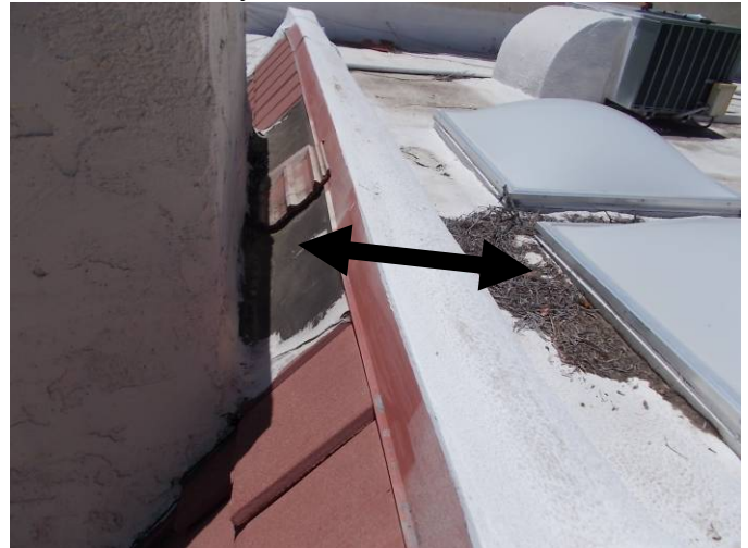
Debris built up by the skylights. The area behind the chimney on the mansard is missing tile.
