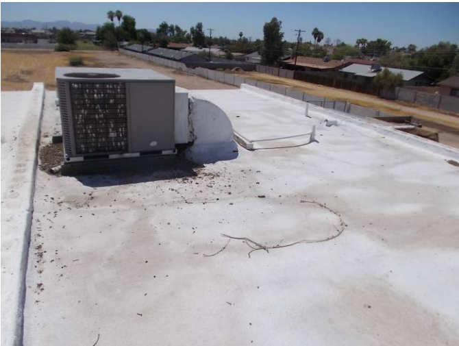
This is an overview of the single layer foam system on 8421 N. 59 th Dr. which is in poor condition.
