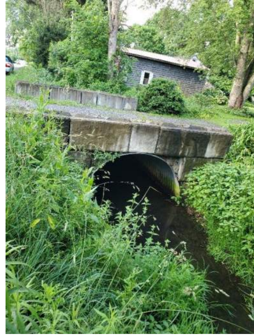
Photo 2.8 – Corrugated Metal Pipe Driveway Culvert
