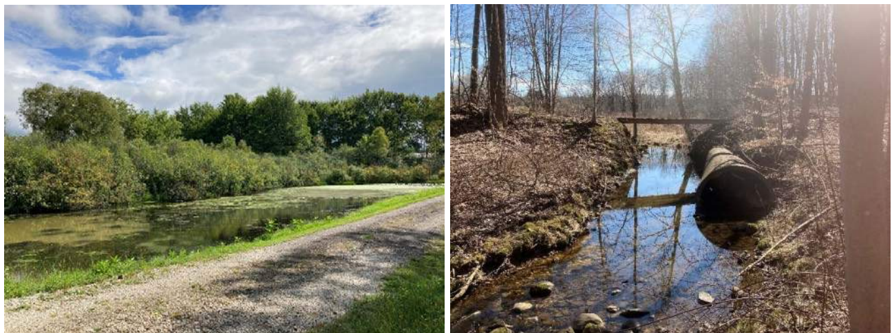
Figure 6. Ponded area upstream of driveway embankment (left) and blown out culvert at old railroad line crossing (right)
