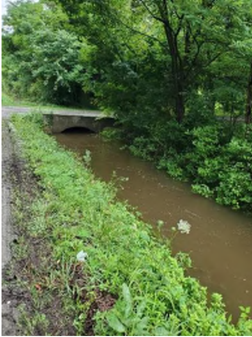
Photo 2.7 – Concrete Driveway Culvert
