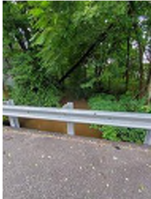
Photo 2.6 – Bridge Guard Rail and West Branch of Black Brook
