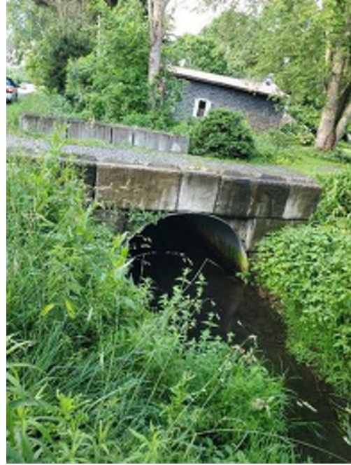
Photo 2.8 – Corrugated Metal Pipe Driveway Culvert
