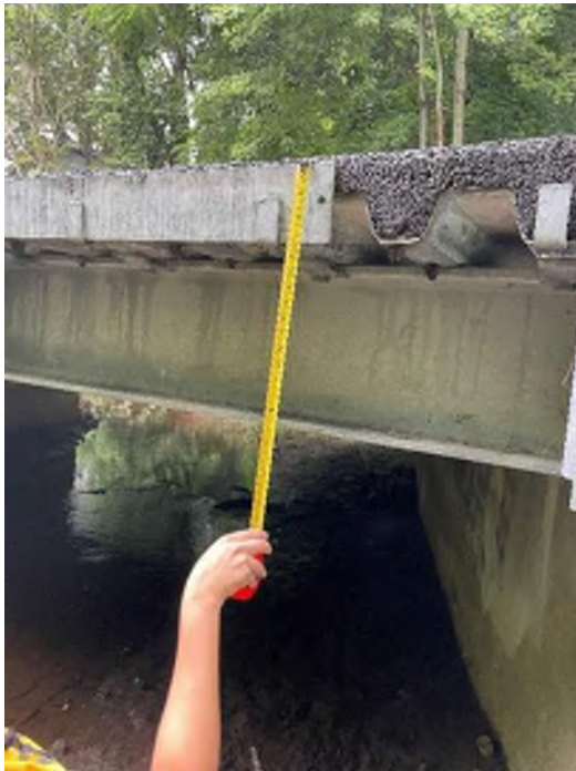
Photo 2.5 – Bridge Girder and Decking
