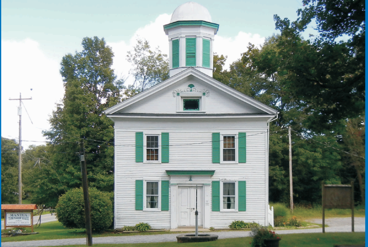
Mantua Township Hall built 1840
