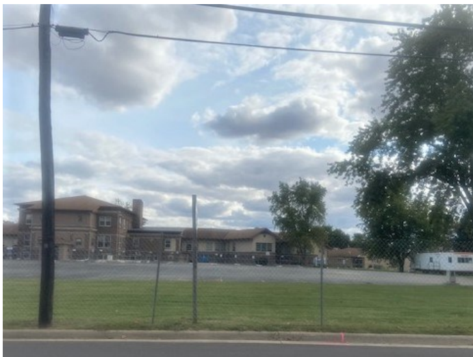
Construction site trailer and fencing go up 10.2020.
