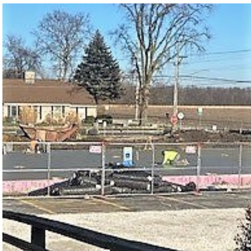
Finishing concrete pad 12.2020.
