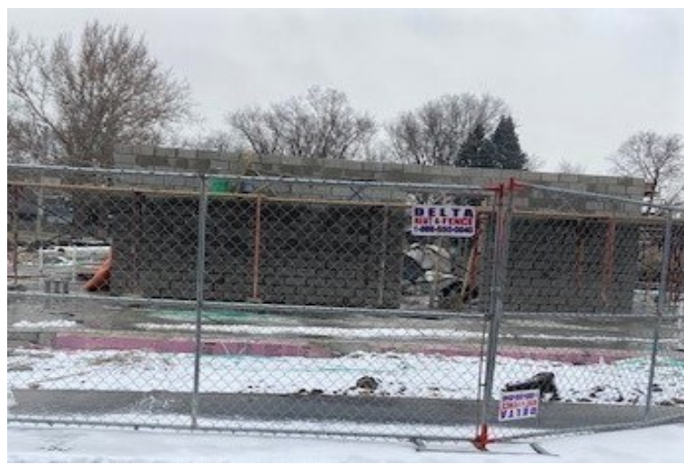
Concrete block conference room/storm shelter built 12.2020.
