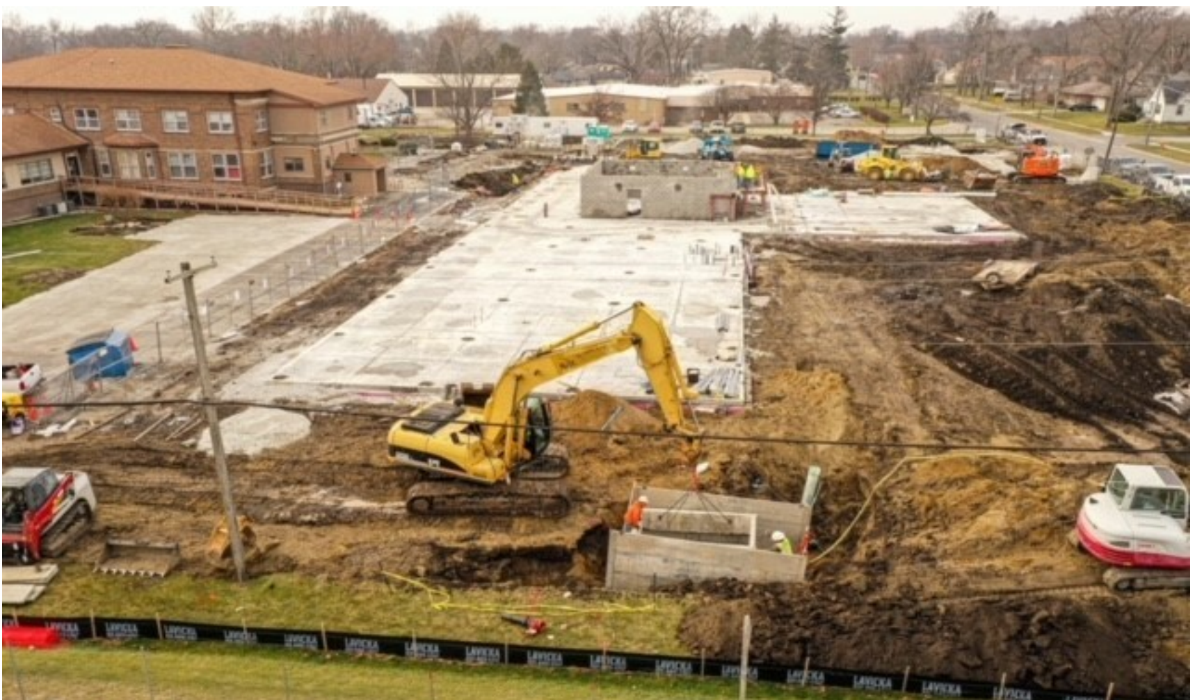
Aerial view of construction site progress 12.2020.
