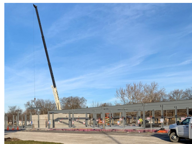
Crane setting metal tresses 12.2020.
