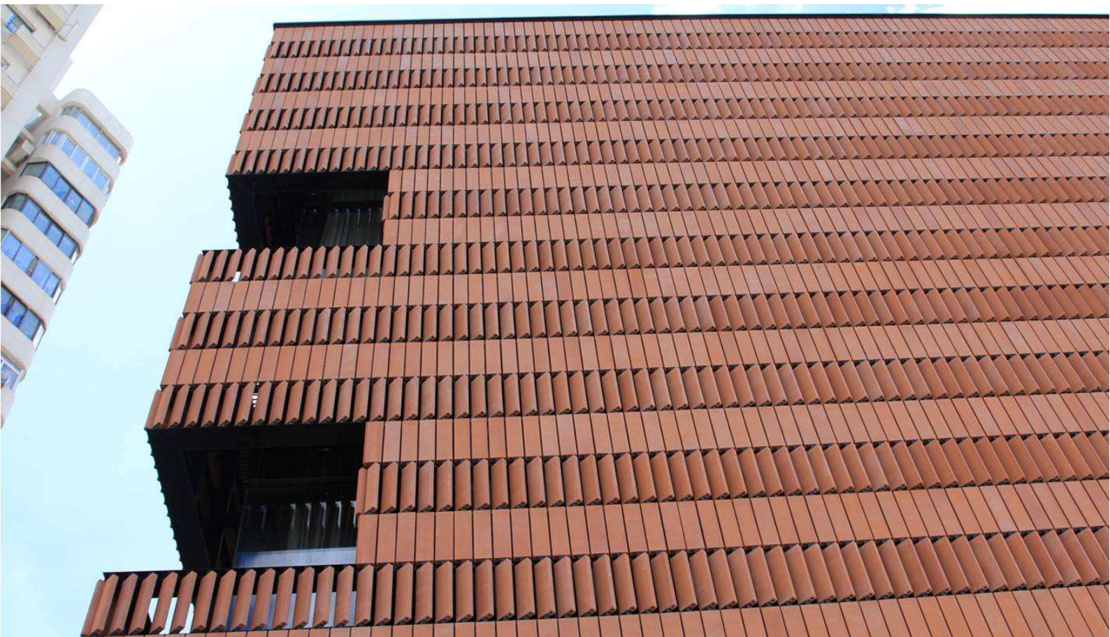
Angled terracotta louvers create a layered facade screen. Shanghai, China.
