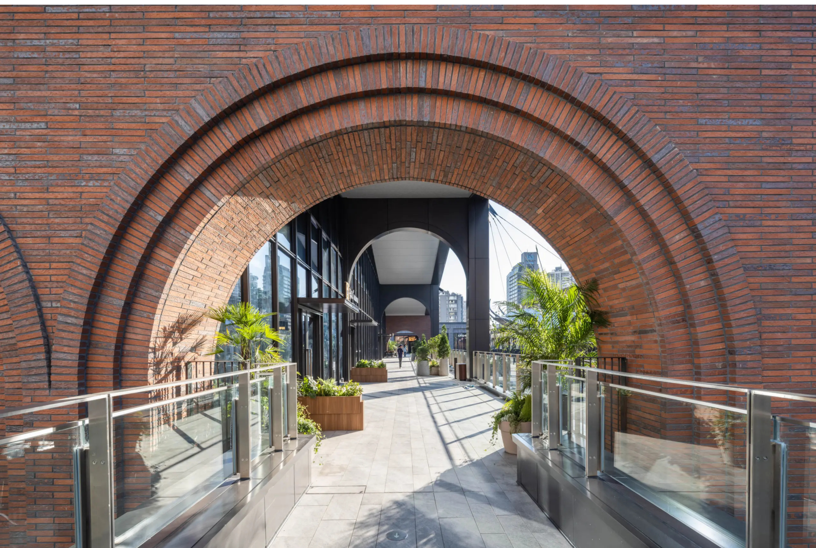
Yiwu Place / Brick arches around a pedestrian passage
