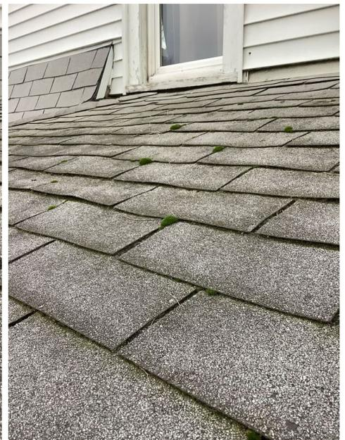
Potential decking failure or Roofed over 2nd layer shingle or moss
