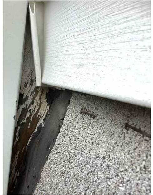
paint or flex n seal the exposed wood
