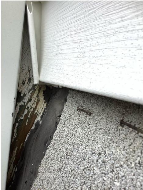
Need roof tar aluminum flashing to keep this protected
