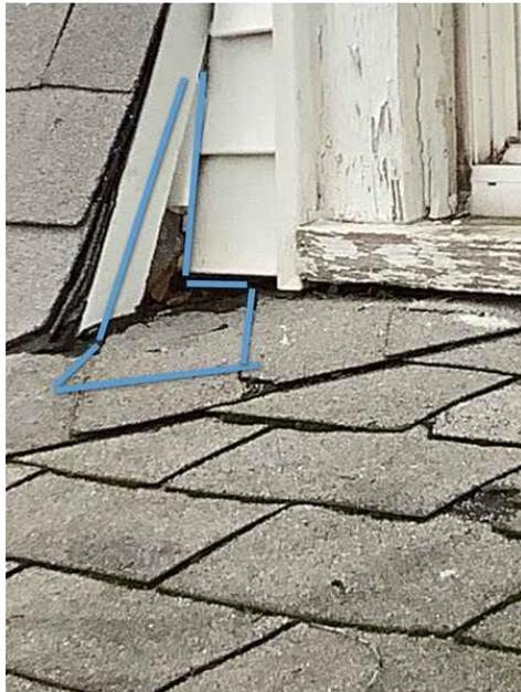
Needs aluminum flashing or caulk at minimum
