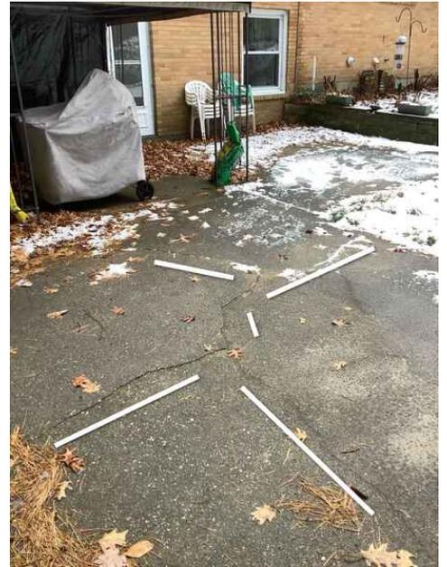
minor cracking, monitor for changes
