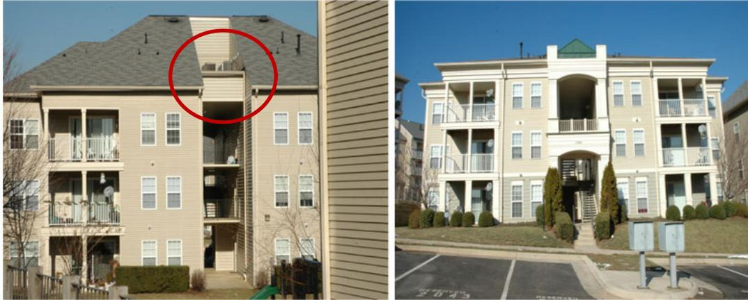
**Figure 73: A concentrated load over the stairwell. Notice it is not evident from the front of the structure.**
