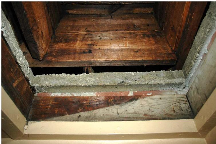
**Figure 9: View from scuttle hole showing layer of concrete ceiling.**
