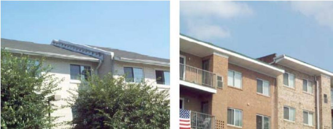
**Figure 24: Exterior clues to the location of a firewall.**
