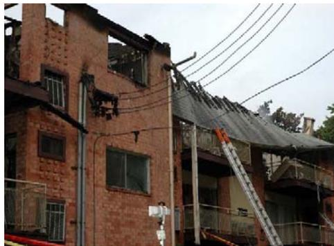
**Figure 72: Attic overhang (soffit) collapse.**
