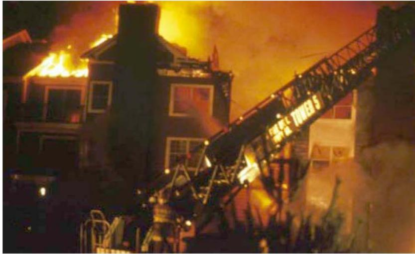
**Figure 38: Light wood frame collapse under fire conditions**
