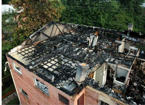
**Figure 71: Gable roof attic fire.**
