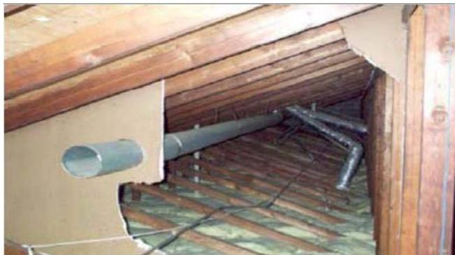
**Figure 23: Breach in firewall/draft stop.**
