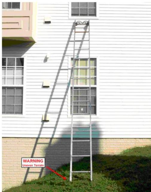
**Figure 89: Ladder on uneven terrain.**
