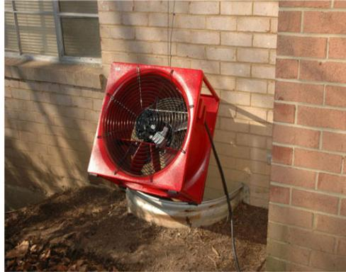
**Figure 91: Venting basement through window well hole.**
