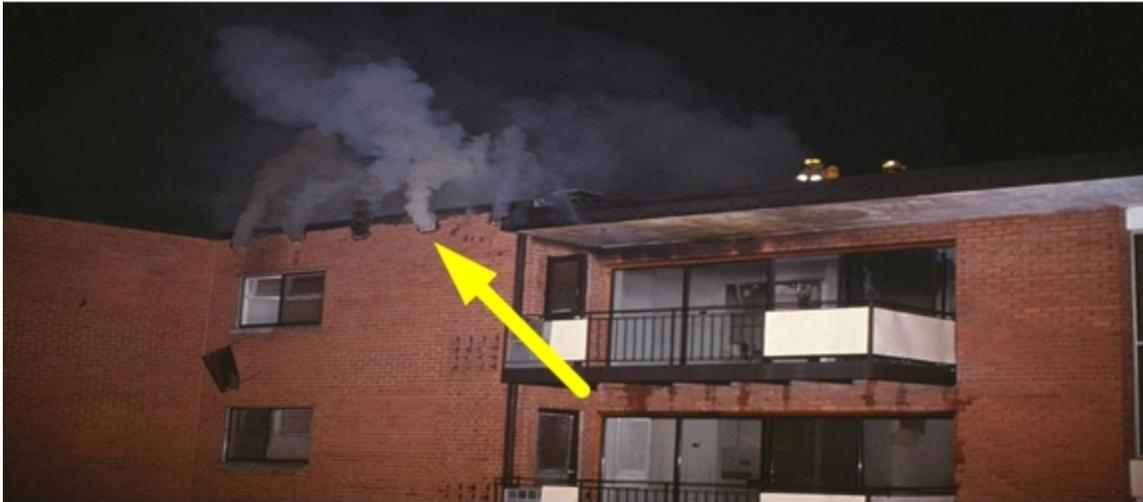
**Figure 70: Smoke showing from the cockloft.**
