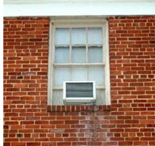
**Figure 17: Window air conditioning unit.**
