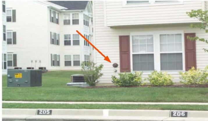
**Figure 34: Sprinkler connection.**
