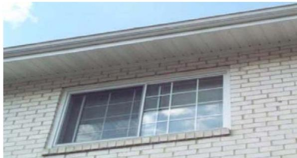
**Figure 21: Example of soffit.**
