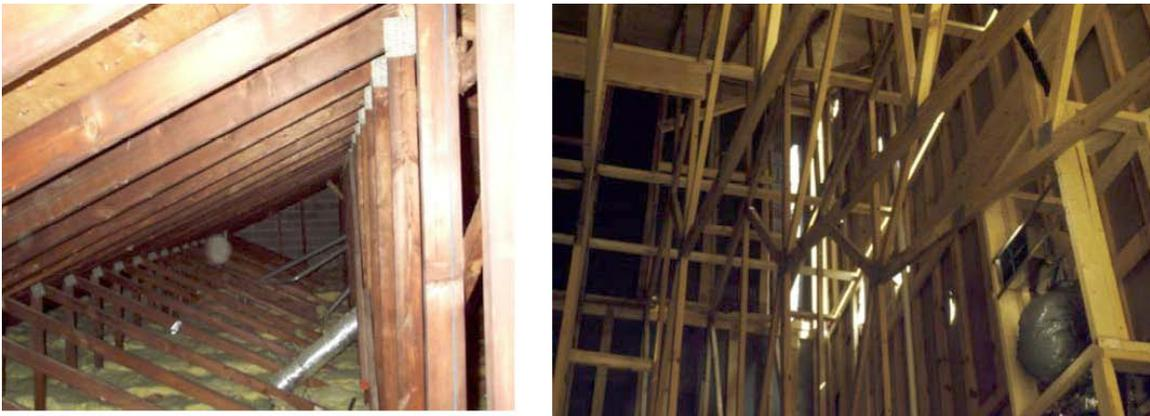
**Figure 19: Common attics from 1960-1970s construction (left) and 1980s to the present construction (right).**
