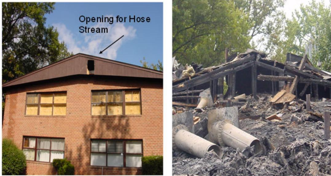
Figure 76: Fire involving a gable roof placed over an existing roof.
