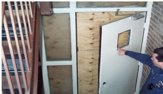
**Figure 80: Terrace-level apartment foyer blocked off from the common stairwell.**
