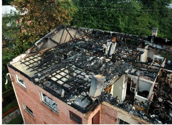
**Figure 71: Gable roof attic fire.**
