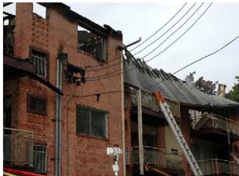
**Figure 72: Attic overhang (soffit) collapse.**
