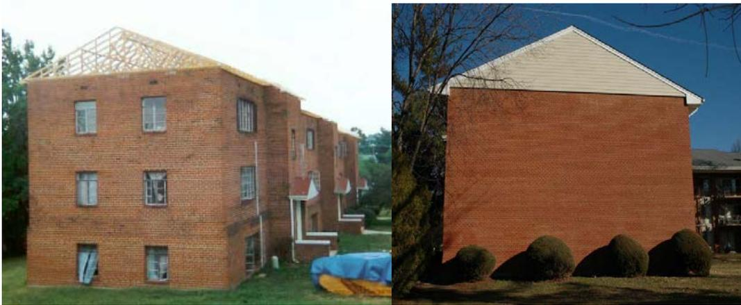
Figure 10: A renovation showing gable over flat roof; vinyl over brick may be an indication of renovation.
