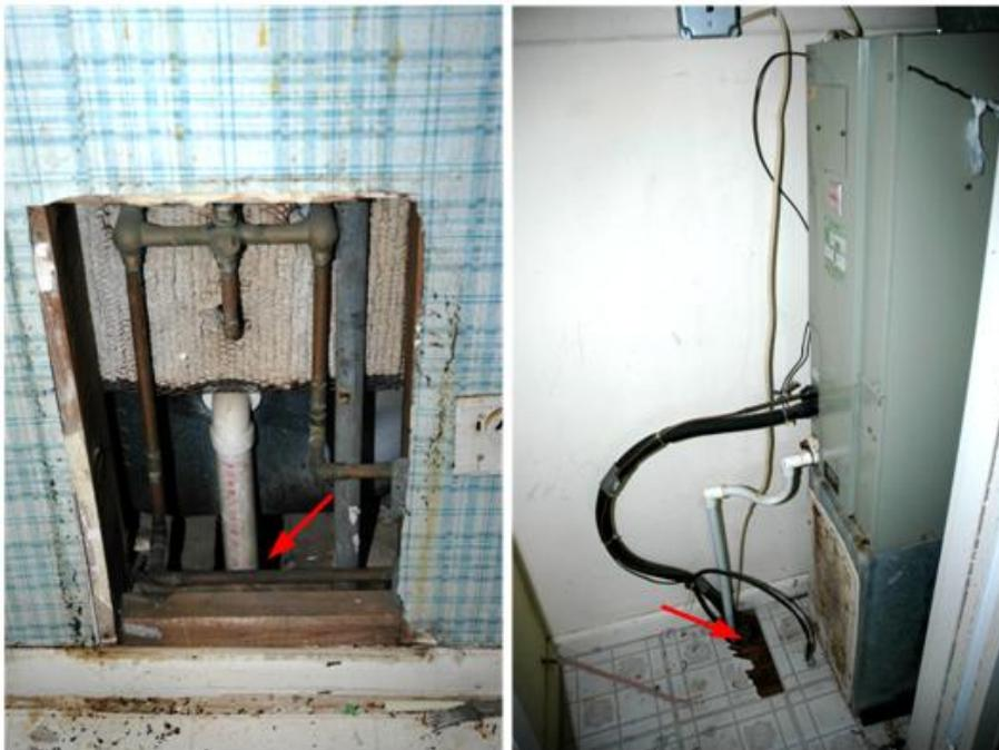
**Figure 88: Examples of plumbing voids.**
