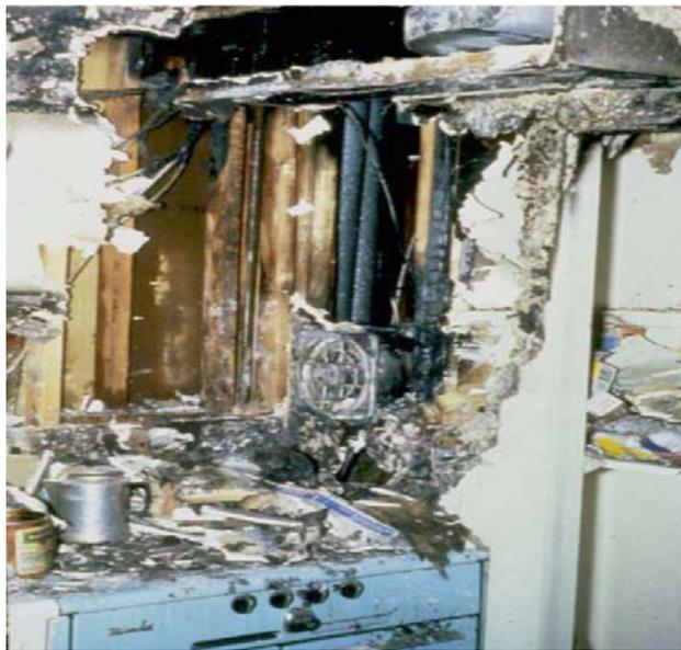
**Figure 39: A minor kitchen fire extends into void space.**
