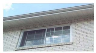
Figure 21: Example of soffit.
