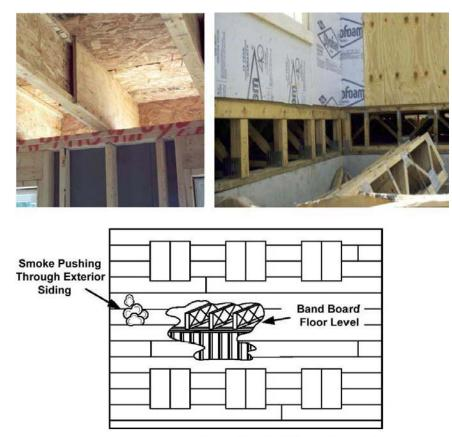
Figure 27: Smoke issuing from the band board area can indicate fire has breached the truss floor space.
