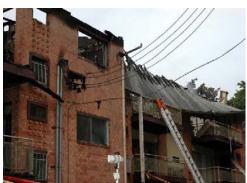
Figure 72: Attic overhang (soffit) collapse.
