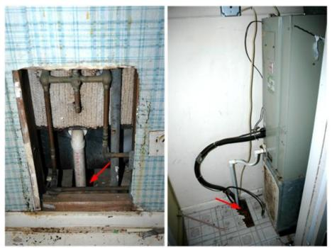
Figure 88: Examples of plumbing voids.
