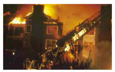
Figure 38: Light wood frame collapse under fire conditions
