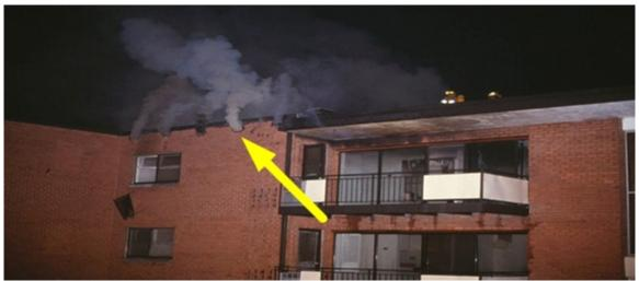
Figure 70: Smoke showing from the cockloft.
