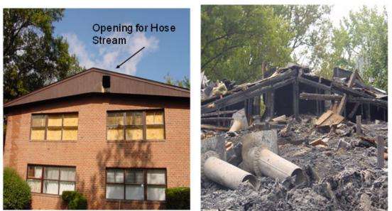
Figure 76: Fire involving a gable roof placed over an existing roof.
