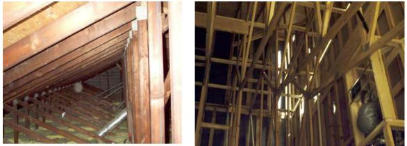
Figure 19: Common attics from 1960-1970s construction (left) and 1980s to the present construction (right).
