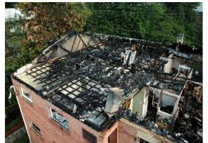
Figure 71: Gable roof attic fire.
