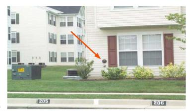
Figure 34: Sprinkler connection.
