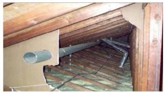
Figure 23: Breach in firewall/draft stop.
