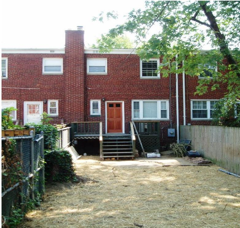
**Figure 5: A rowhouse is a multi-story dwelling attached to at least two other dwellings. These dwellings may or may not be separated by fire walls. Typically a rowhouse will have a common cockloft under a flat roof. The figure shows the rowhouse from Side Alpha (top), and Side Charlie (bottom).**
