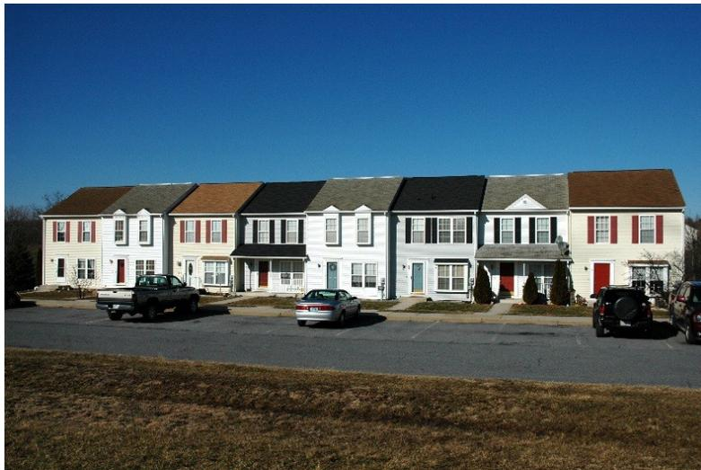
**Figure 1: A townhouse is a multi-story dwelling normally attached to several other units. Typically, adjacent occupancies have rated floor and wall assembly separation. Townhouses most often will have an attic with a pitched roof.**
