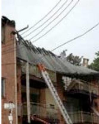
**Figure 21: Attic overhang (soffit) collapse.**
