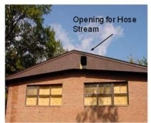
Figure 24: Opening into an attic for a hose stream.
