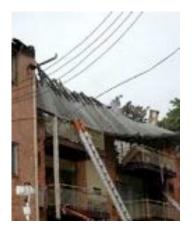
Figure 21: Attic overhang (soffit) collapse.
