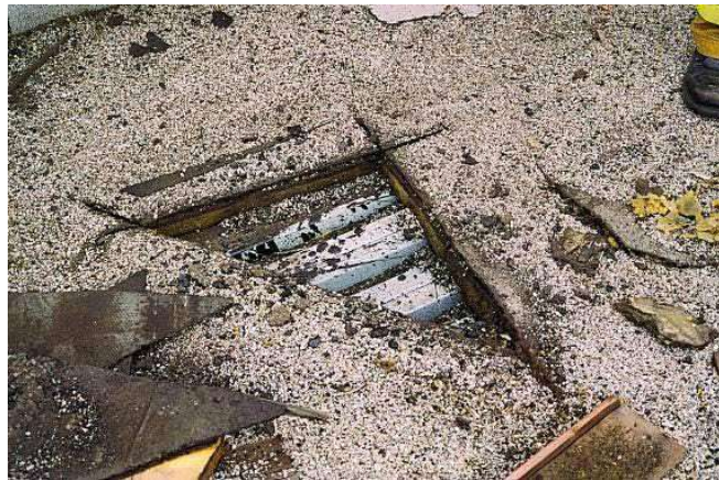
Figure 28. Inspection holes.
