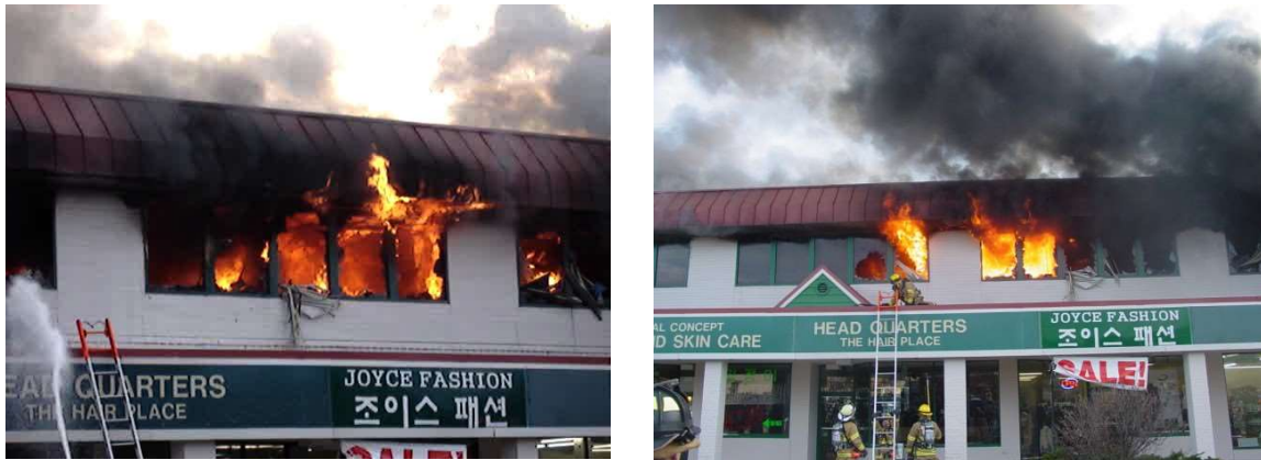
Figure 24. Fire extension via the front wall facade.
