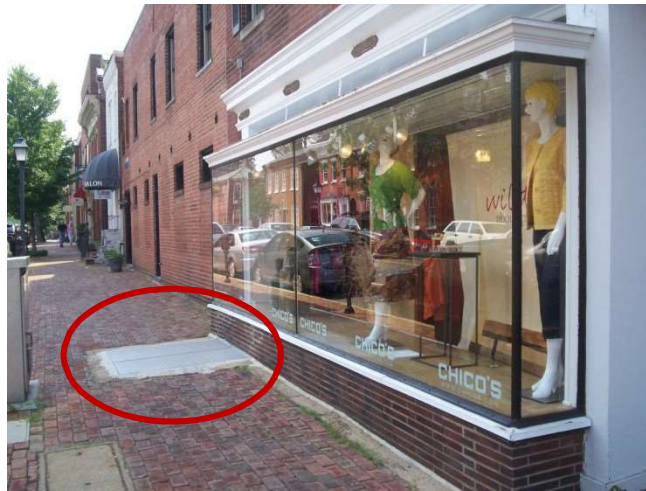
Figure 17. Basement entrance in sidewalk.
