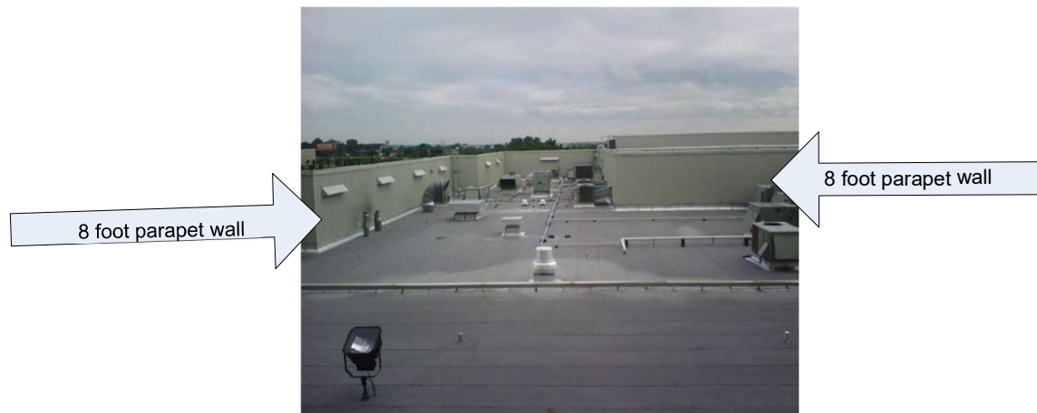
Figure 14. Parapet walls on roof edge.
