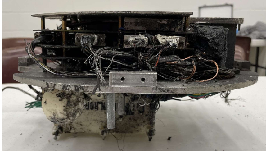
Figure 30 - Electrical system after recovery, side view
