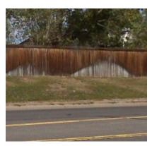
Water is one of the most damaging elements for a fence and leads to a shorter lifespan. Irrigation systems run often, which discolors the fence and causes the wood to rot much sooner than it would naturally. The ground around the posts also gets saturated, which causes the posts to rot and even break off at the ground.
