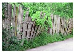
Most species of vines are likely to be treacherous to a wood fence's longevity. The rotting, cracking, twisting, moisture transfer, and other structural damage that vines can cause to your wooden fence mean that most species should be kept away.
