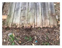
Rot is an ever-present threat to the health of your fence and is caused by the wood's prolonged exposure to moisture, mainly via contact with the soil. Rot will weaken the fence's structural integrity and dramatically reduce its lifespan.
