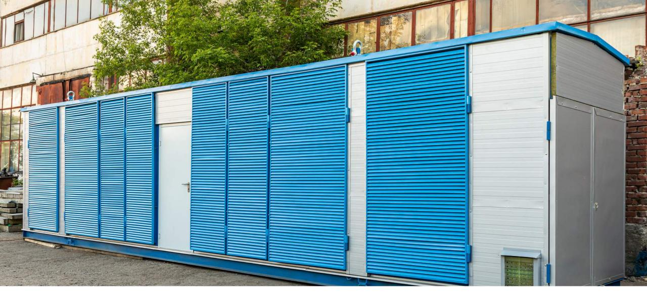
Materials, heat resistance – the Smartbox is made of sandwich panels
