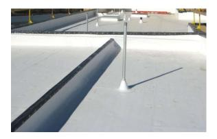
Short for thermoplastic polyolefin, TPO is a single-ply roofing membrane that offers excellent performance at a cost-effective price. Heat-welded seams provide superior strength. TPO's long-term heat, UV, and natural fungal resistance, plus flexibility without need for plasticizers also make TPO a reliable low-slope roofing system.
