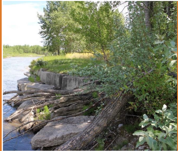
Example of an altered streambank that is a candidate for a soil bioengineering bank stabilization project to improve cover and root mass protection from native tree and shrub species and to remove concrete rubble.
