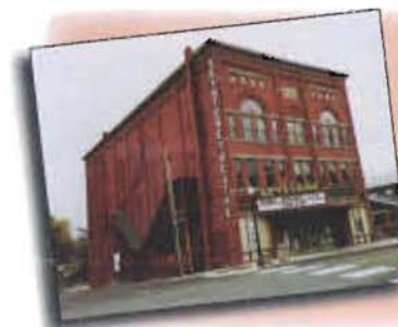
#15 601 Main St., Keystone Theatre, Romanesque Revival, 1886. Originally the Hale Opera House where John Phillip Sousa's Band performed. First floor once a railroad station for Southern and New York Railroad. In 1913 renamed and transformed into present 'movie house'.
