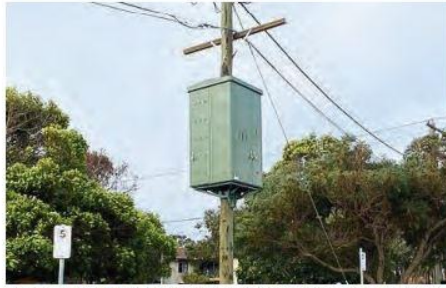
Batteries mounted on the top of power poles are like virtual power plants and could supply local energy to smaller towns like Newhaven or Smiths Beach.
