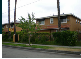
FULTON AVE North Hollywood 12 Units
