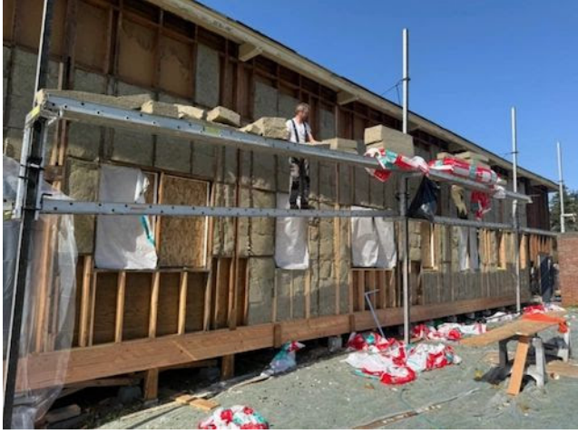
Reframed insulation going up
