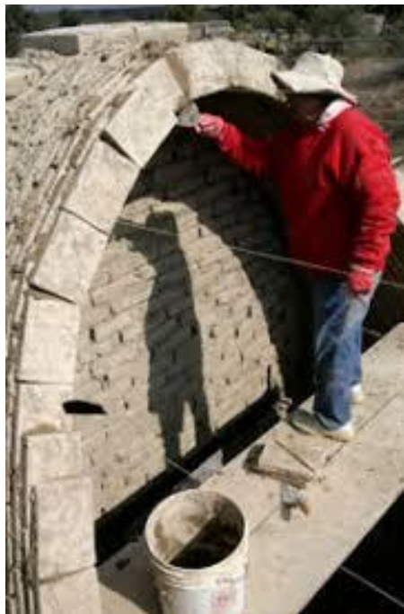
Figure 6: Students building the wall.
