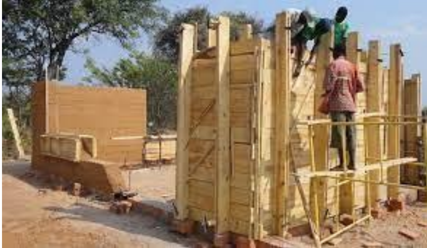
Figure 7: The use of wooden forms to build rammed earth walls
