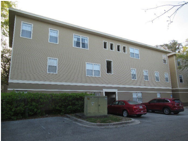
Exterior building overview
