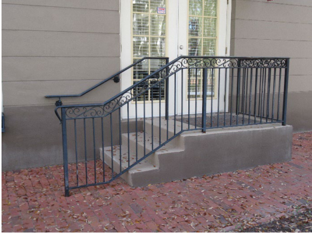
Metal railing at Building O entry
