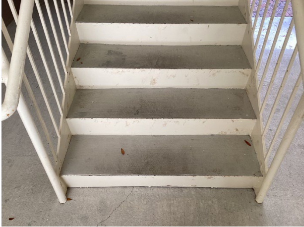
Metal staircase with concrete treads
