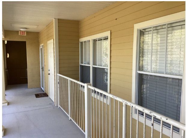
Fiber cement siding at breezeway
