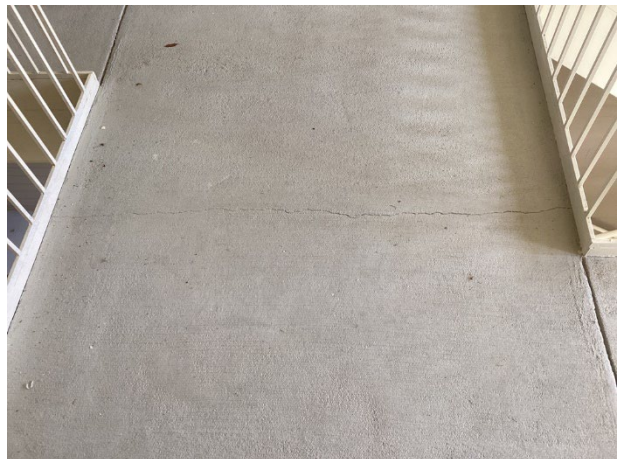
Concrete cracks
