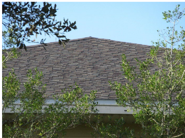
Asphalt shingle roof
