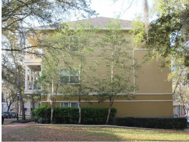
Asphalt shingle roof
