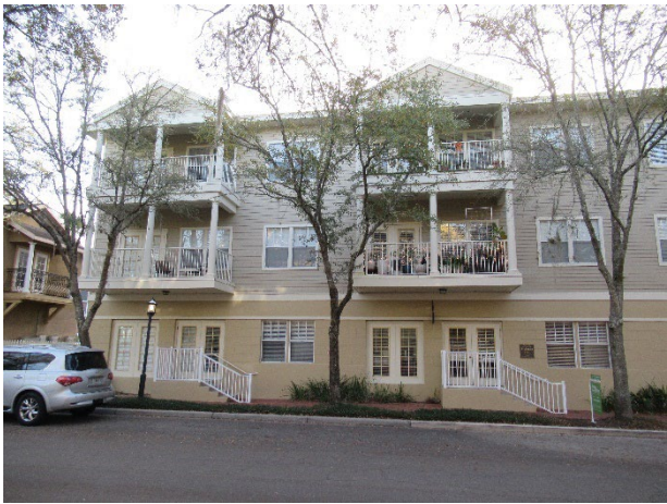
Exterior building overview
