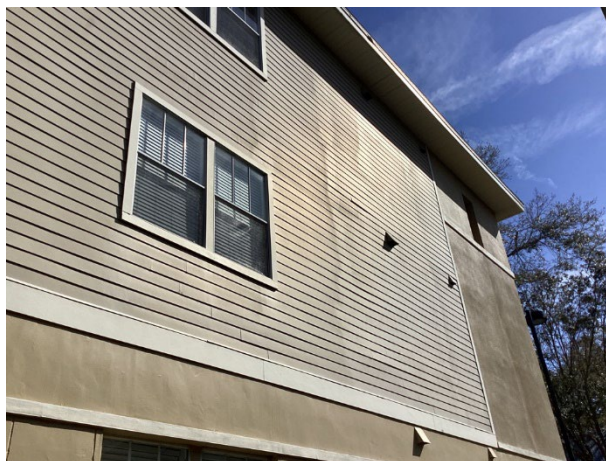
Fiber cement siding overview
