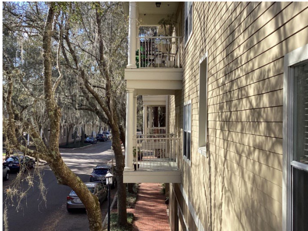
Balcony overview with concrete surface
