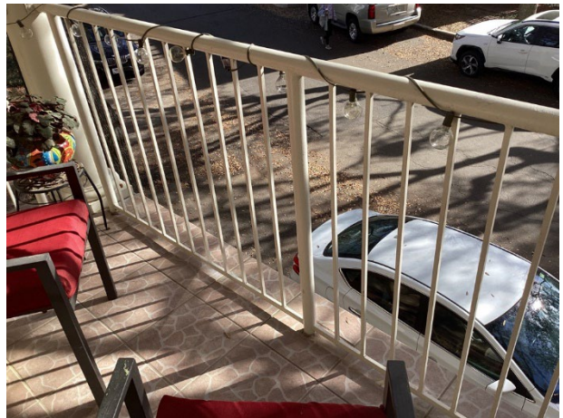
Metal railing at balcony
