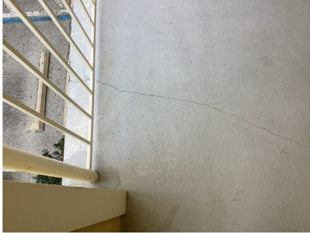
Concrete cracks
