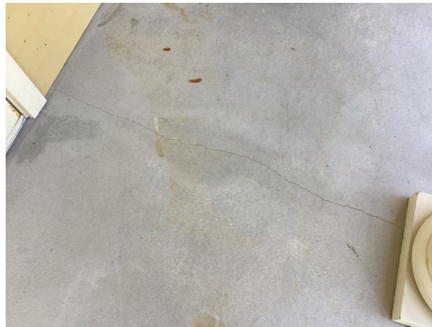
Concrete cracks
