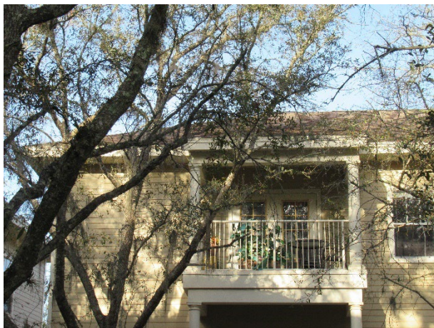
Asphalt shingle roof
