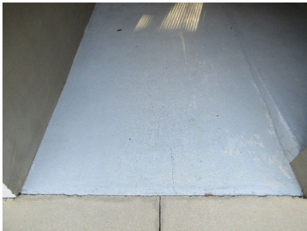
Concrete cracks
