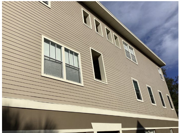
Fiber cement siding overview
