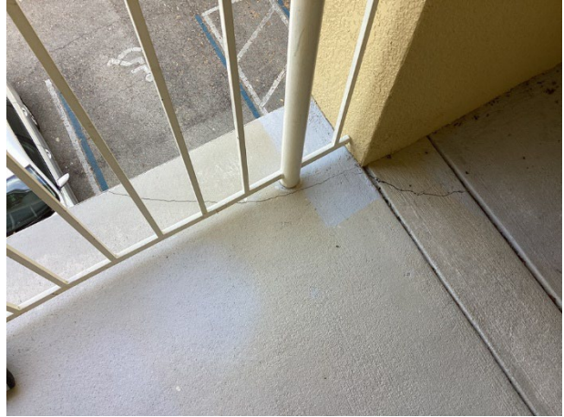
Concrete cracks
