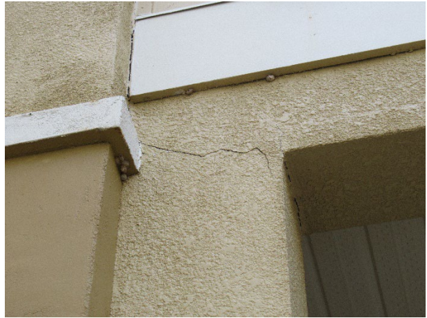
Stucco crack
