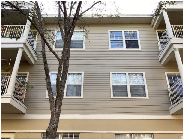
Fiber cement siding overview
