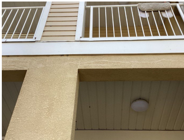
Stucco cracks
