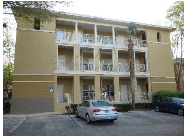
Exterior building overview
