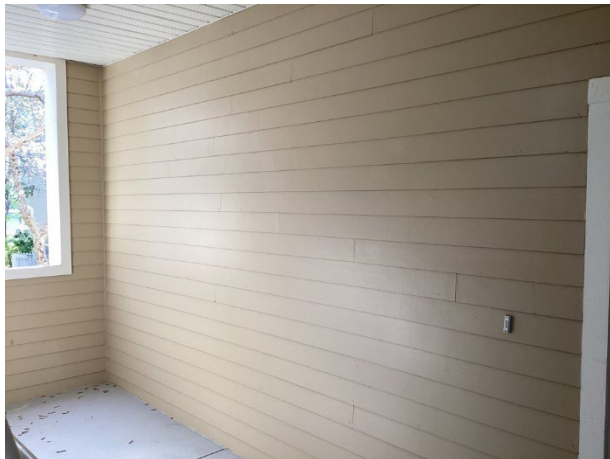
Fiber cement siding at breezeway
