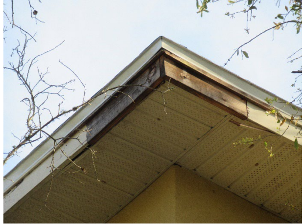
Fascia board repair
