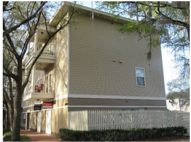
Exterior building overview
