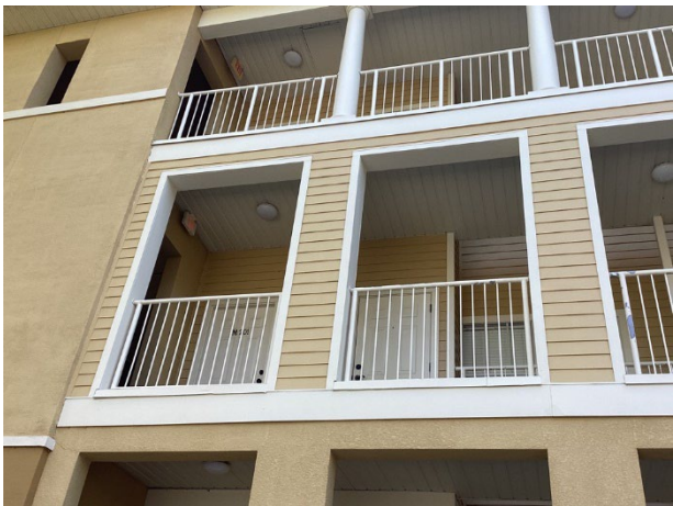
Metal railings at breezeways
