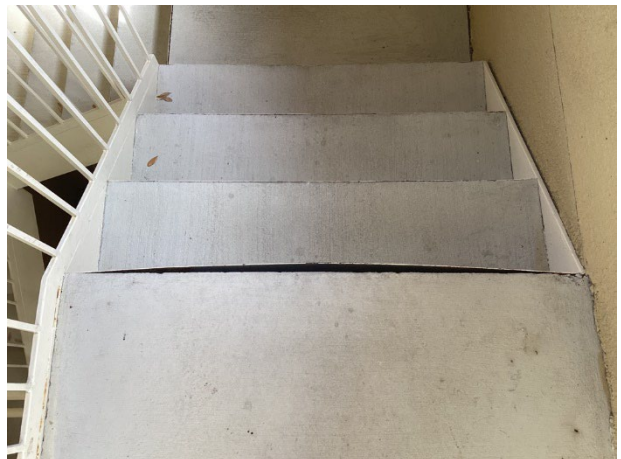
Metal frame damage
