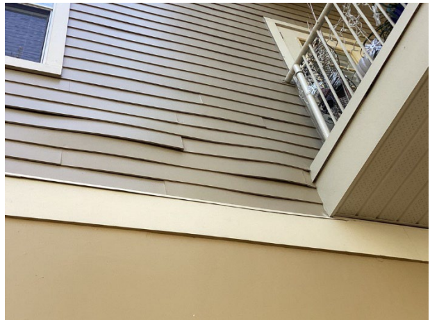
Siding damage
