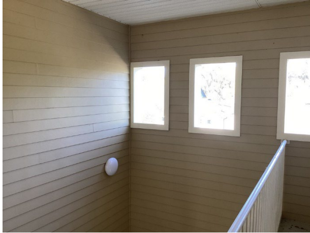
Fiber cement siding at breezeway
