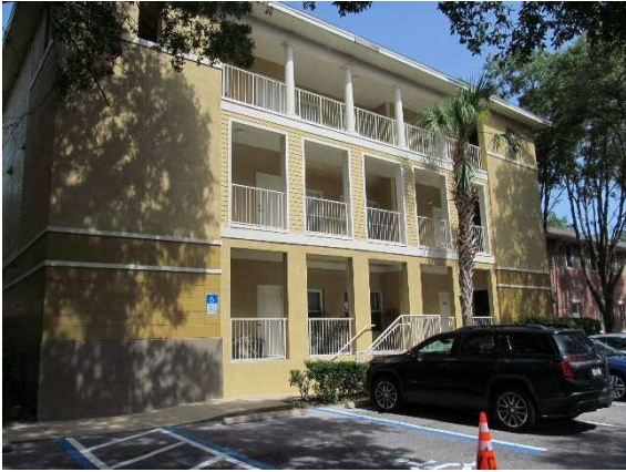
Building M rear view
