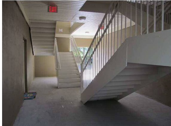
Building Q central stairs common area
