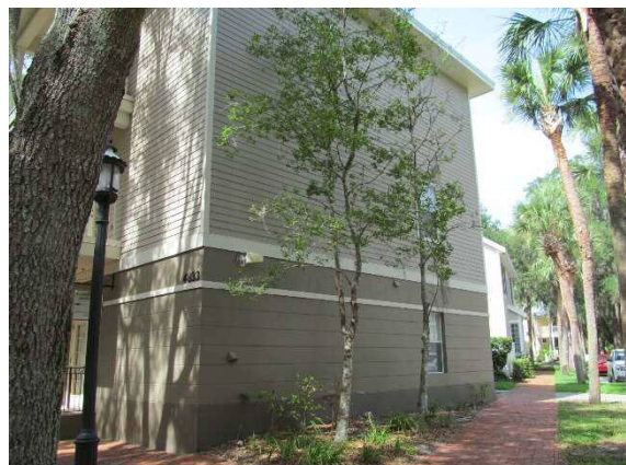
Building O side view
