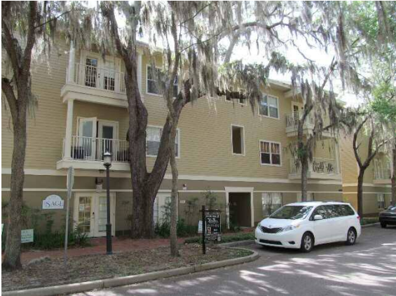
Building P front view
