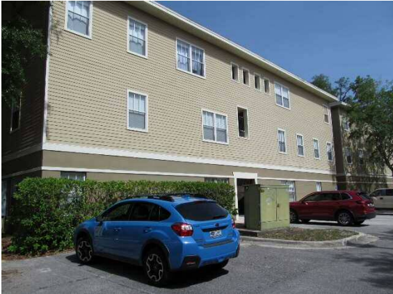
Building Q rear view
