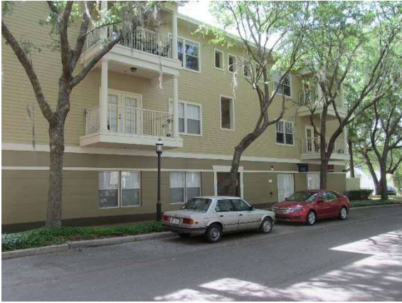
Building Q front view
