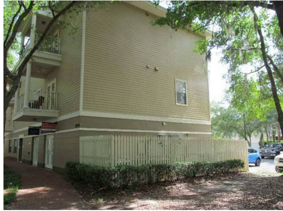
Building Q side view
