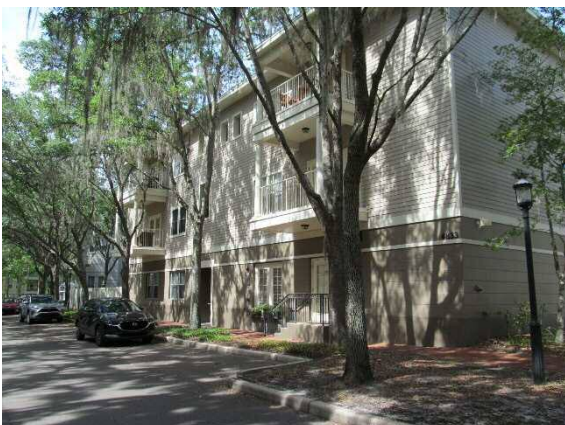
Building O front view
