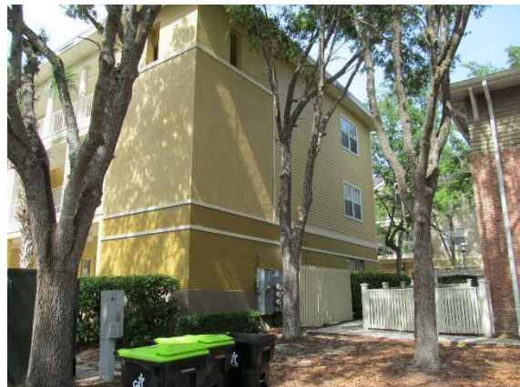
Building M side view
