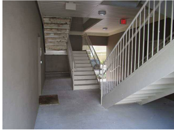
Building O central stairs common area
