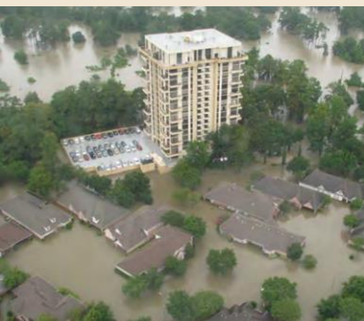
Flooding of Cypress Creek near Champions Forest Drive. Hurricane Harvey. Photo Credit: HCFCD.
